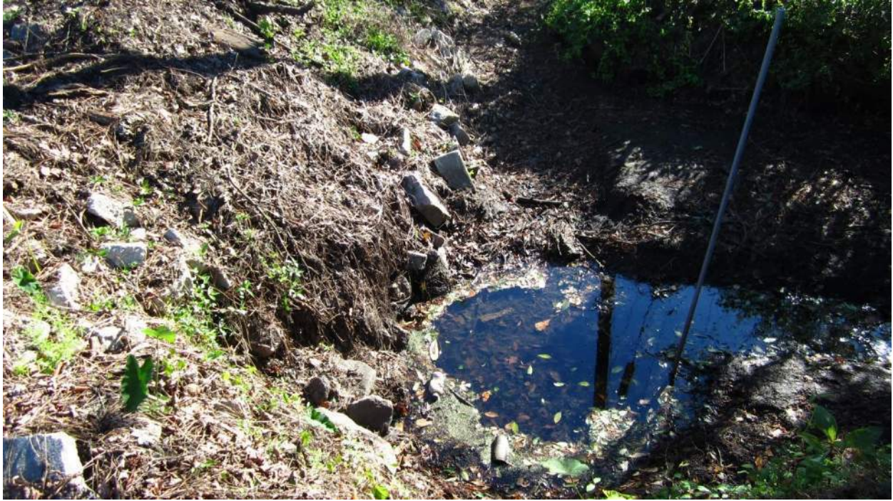
Buried inlet end of First Boulevard 30-inch RCP crossline pipe
