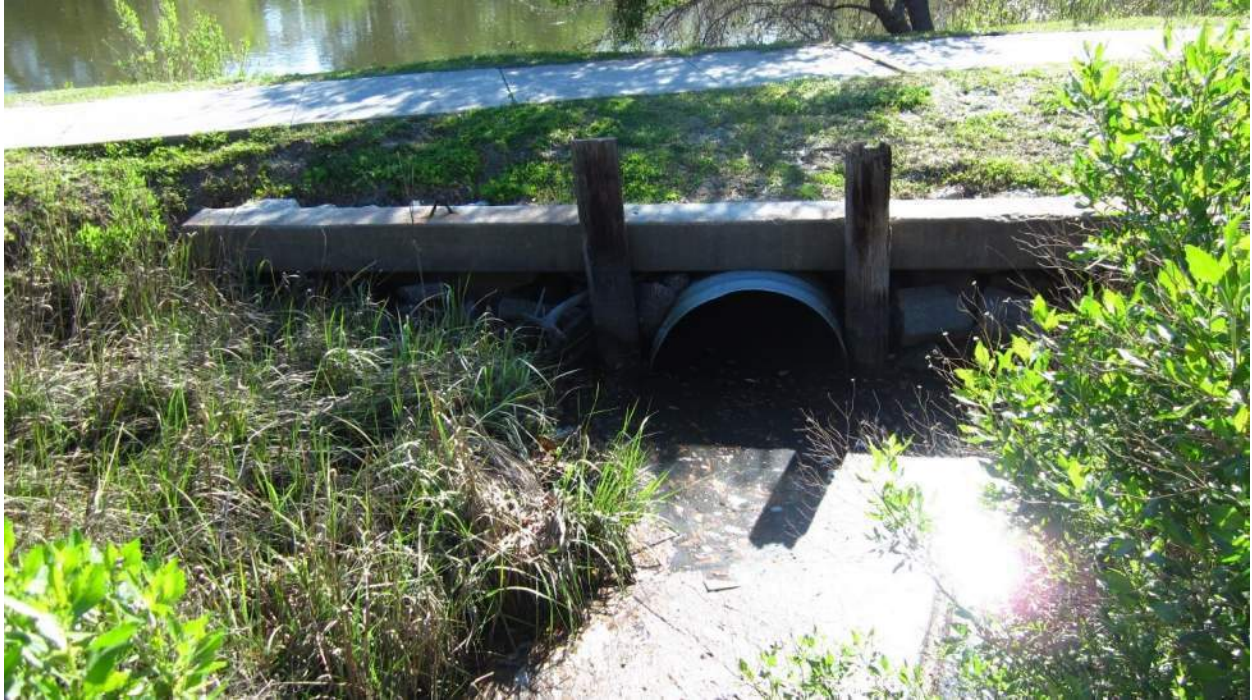
Duck Pond 36-inch CMP outlet pipe
