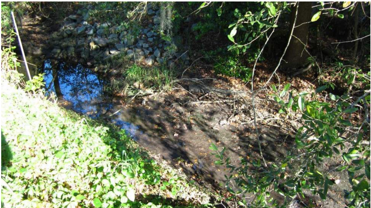
Sideline ditch along First Boulevard, upstream of Jane Way crossing
