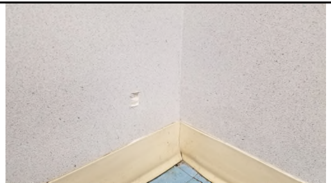
Picture 10 – *HA20 Sheetrock Walls
