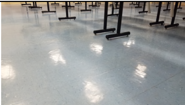
Picture 9 – Blue 12x12 Floor Tiles w/Mastic (Not Included in Scope of Renovation)
