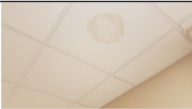
Picture 15 – *HA30 2x2 Textured Ceiling Tiles
