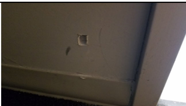
Picture 11 – *HA20 Sheetrock Walls
