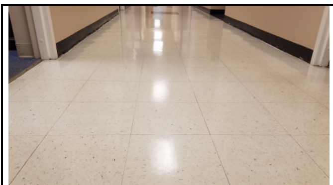
Picture 5 – White 12x12 Floor Tiles w/Mastic (Not Included in Scope of Renovation)
