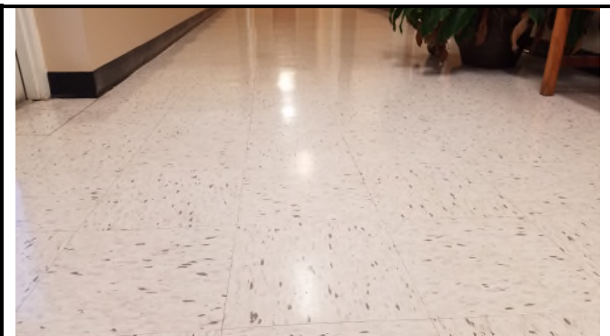
Picture 4 – White 12x12 Floor Tiles w/Mastic (Not Included in Scope of Renovation)
