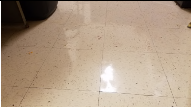
Picture 7 – Beige 12x12 Floor Tiles w/Mastic (Not Included in Scope of Renovation)
