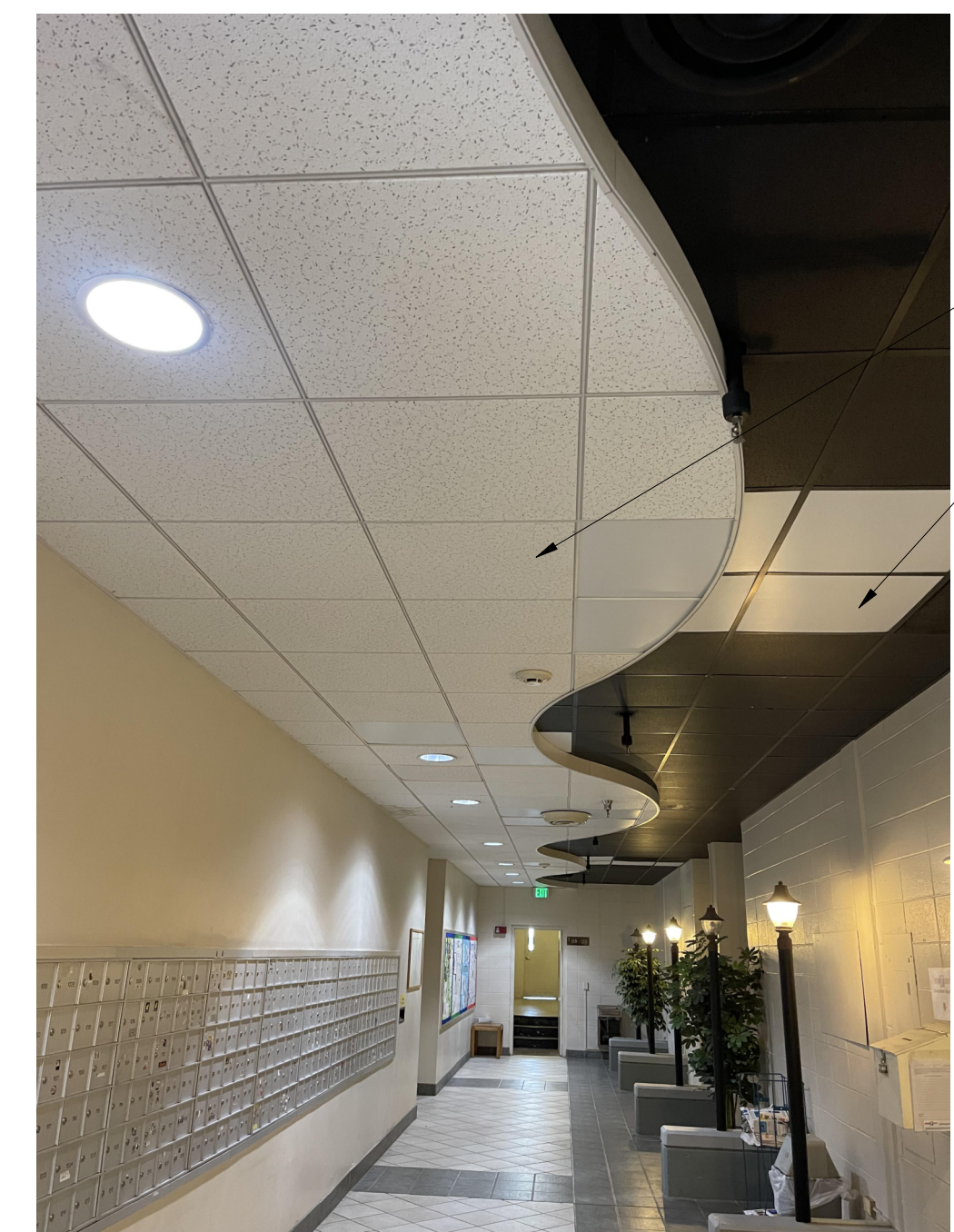
B: Existing Corridor 152 ceiling.
