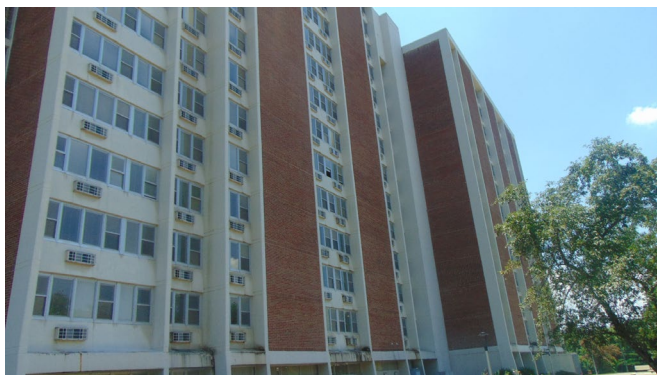
Building - Side C
