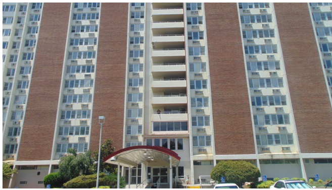
Building - Side A
