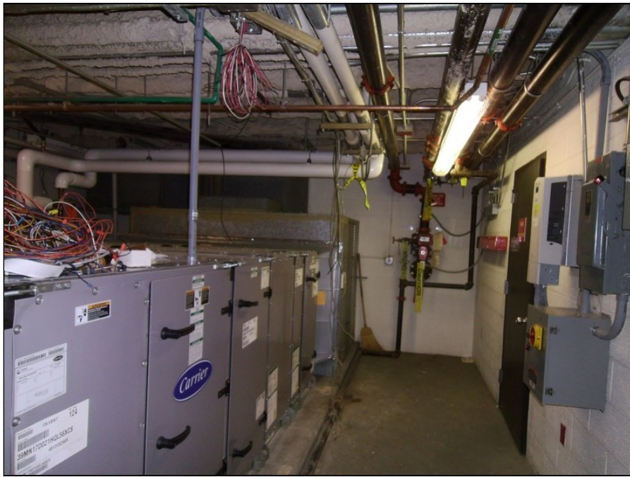
11 - View of basement electrical mechanical room.
