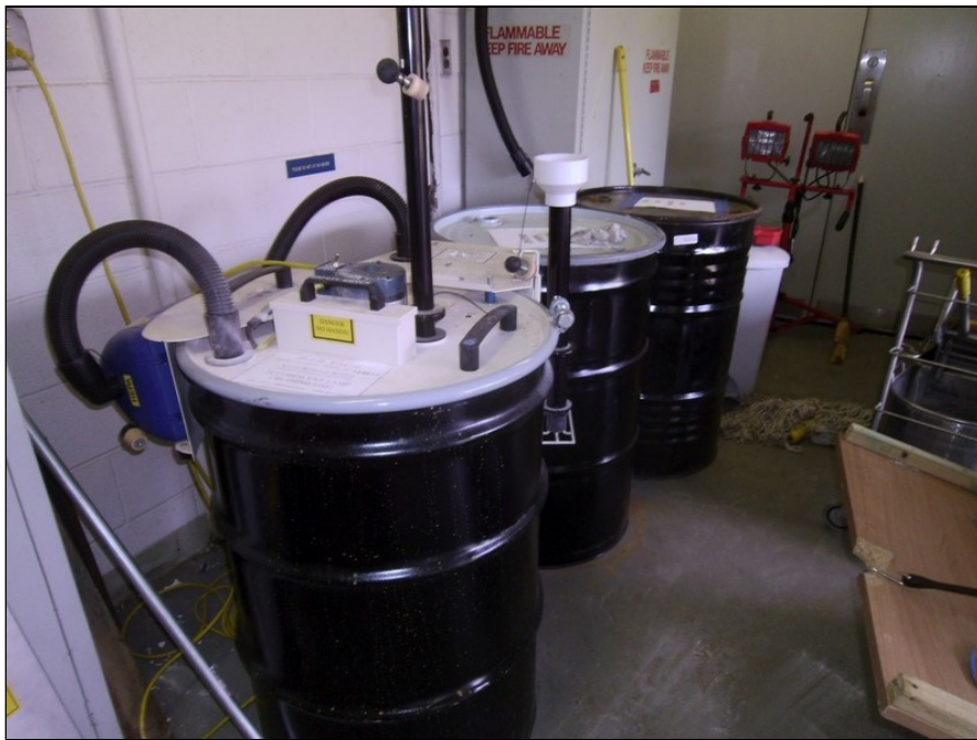
16 - View of fluorescent lamp disposal/recycling drums within basement area.
