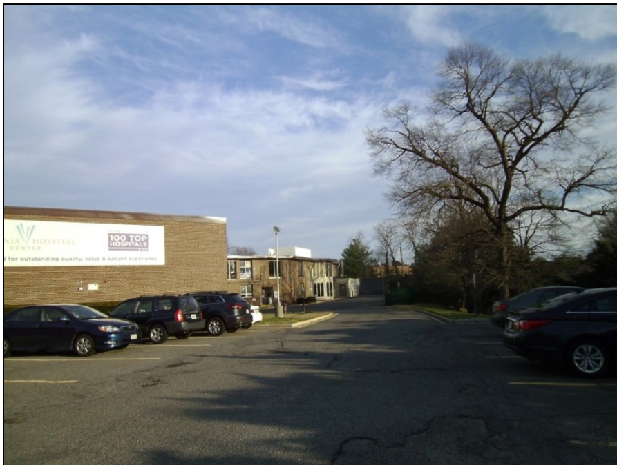
4 - View of west service entrance
