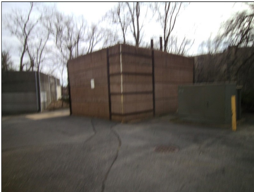
10 - View of Generator 3 area.
