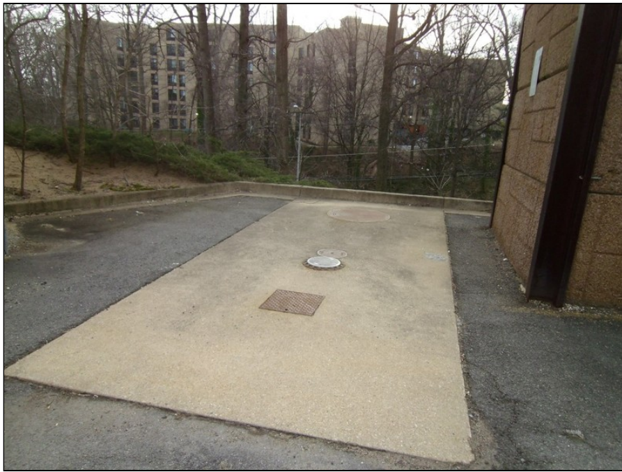
9 - View of Generator 3 UST area.
