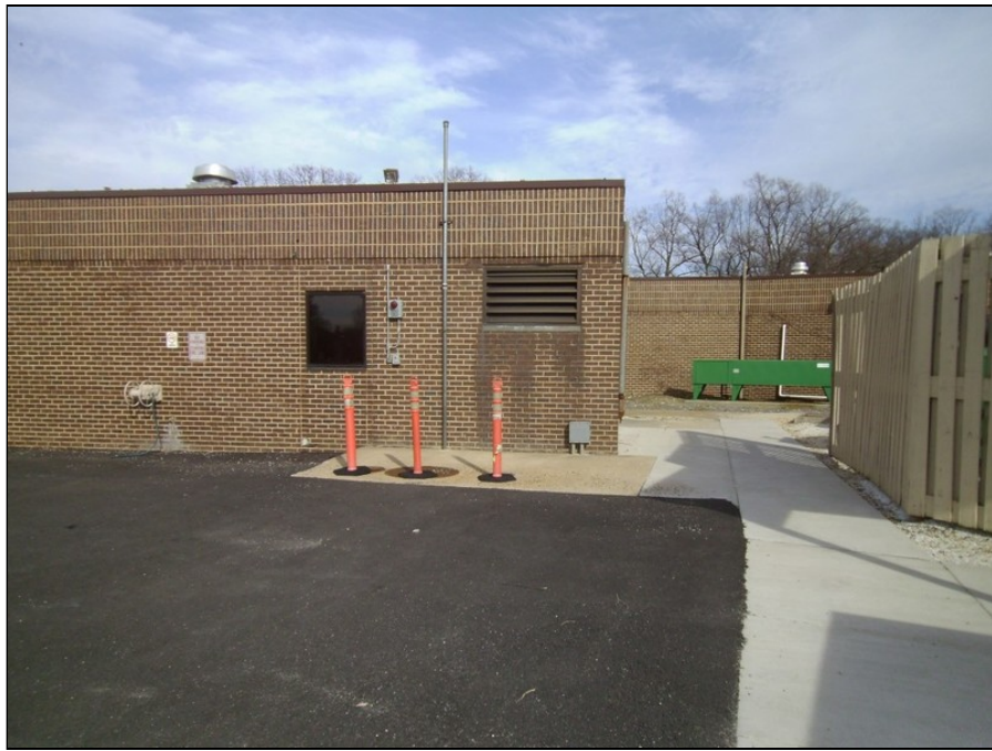
7 - View of Generator 1 & 2 UST area.
