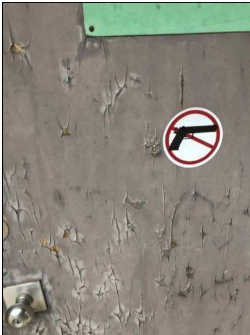
10 - View of Lead Based Paint on a Brown Metal Door. XRF Reading No. 1056.
