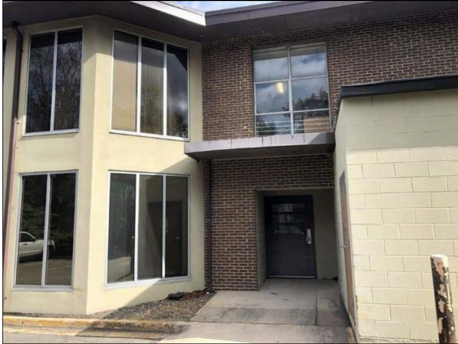
11 - View of Lead Based Paint on a Brown Metal Door. XRF Reading No. 1077.
