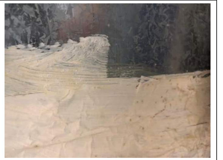
Photo #56 Material: White Duct Seam Sealant On Metal Sample Result: No Asbestos Detected
