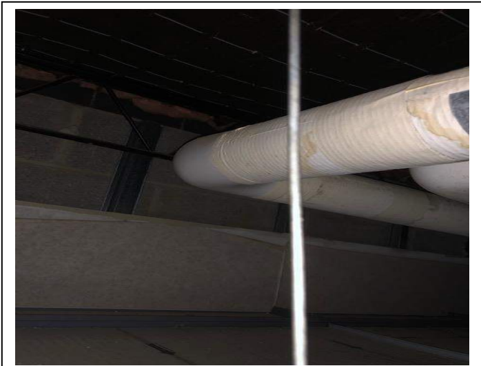
Photo #19 Material: White Pipe Seam Sealant (New) Sample Result: No Asbestos Detected
