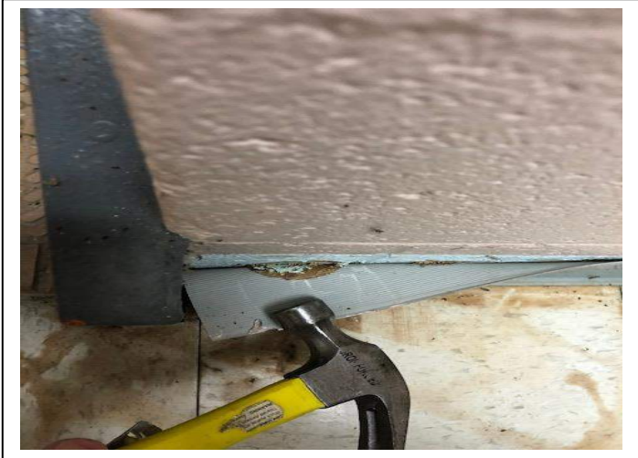
Photo #9 Material: Tan Baseboard Mastic Sample Result: No Asbestos Detected
