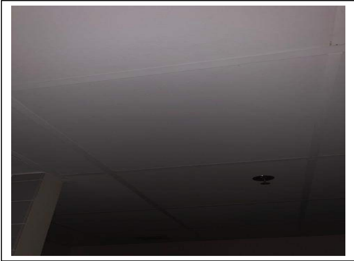
Photo #21 Material: 2'x4' Smooth Ceiling Tile Sample Result: No Asbestos Detected
