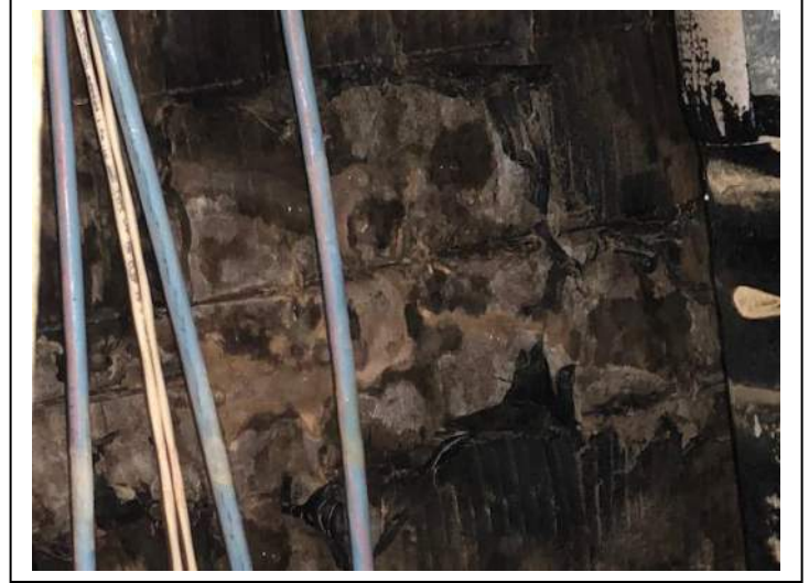
Photo #82 Material: Cement Paper Support Sample Result: No Asbestos Detected
