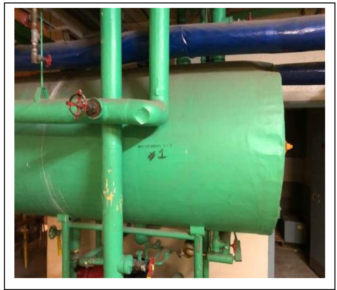
Photo #34 Material: Green Canvas Tank Sample Result: No Asbestos Detected
