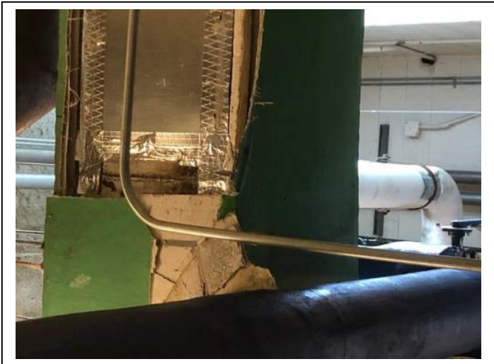
Photo #23 Material: Green Canvas Mudded Duct Sample Result: No Asbestos Detected
