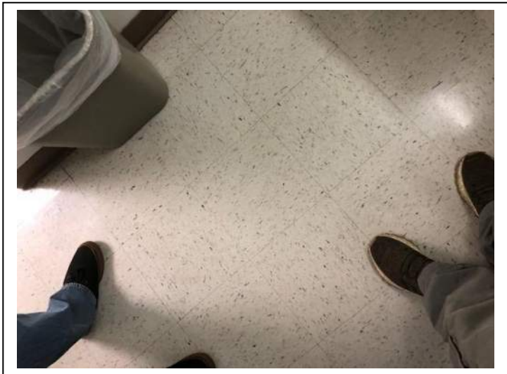
Photo #68 Material: 12"x12" White with Black Specks Sample Result: No Asbestos Detected
