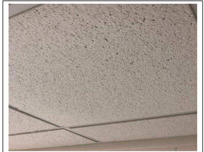
Photo #16 Material: 2'x2' Rough Ceiling tile Sample Result: No Asbestos Detected
