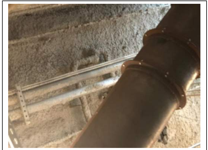
Photo #24 Material: Spray Applied Fire Proofing Sample Result: No Asbestos Detected
