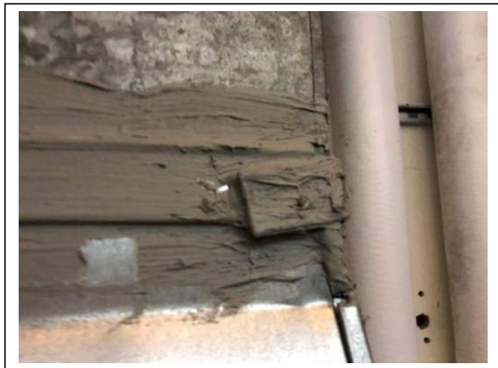
Photo #43 Material: Gray Metal Duct Seam Sealant Sample Result: No Asbestos Detected
