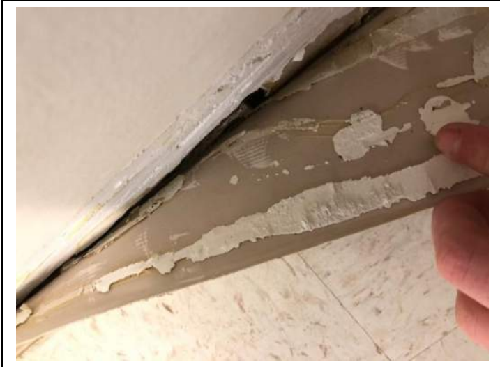
Photo #53 Material: White Baseboard Mastic Sample Result: No Asbestos Detected
