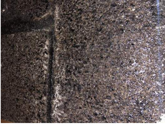
Photo #69 Material: Black Vapor Barrier Sample Result: No Asbestos Detected
