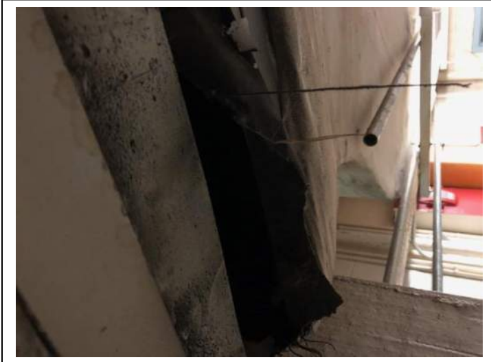
Photo #37 Material: Cloth Vibration Dampner Sample Result: No Asbestos Detected
