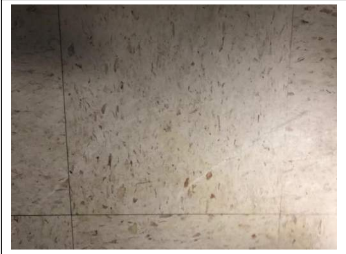
Photo #17 Material: 12"x12" White With Red Specks Floor Tile Sample Result: No Asbestos Detected
