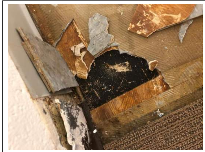
Photo #47 Material: 12"x12" Tan Floor Tile Sample Result: No Asbestos Detected
