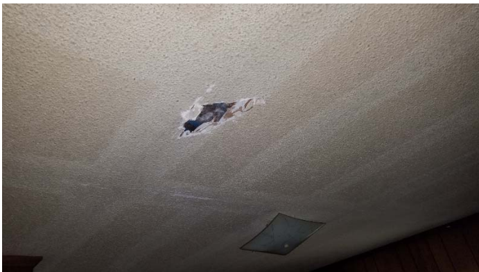
Photo 5 – Popcorn ceiling texture in left rear bedroom.
