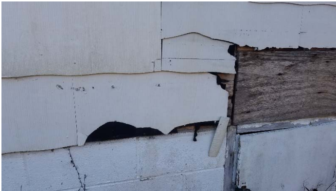
Photo 3 – Transite exterior siding with black felt.
