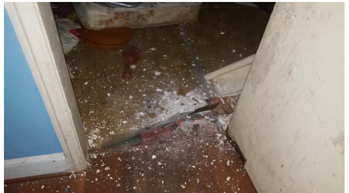
Photo 10 – Kitchen flooring layers.
