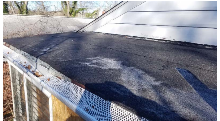
Photo 4 – Back porch roof.
