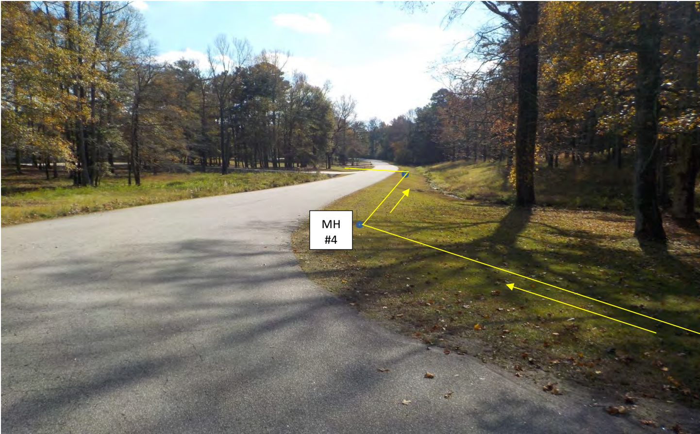
MH #5 to MH #4 to MH #3
