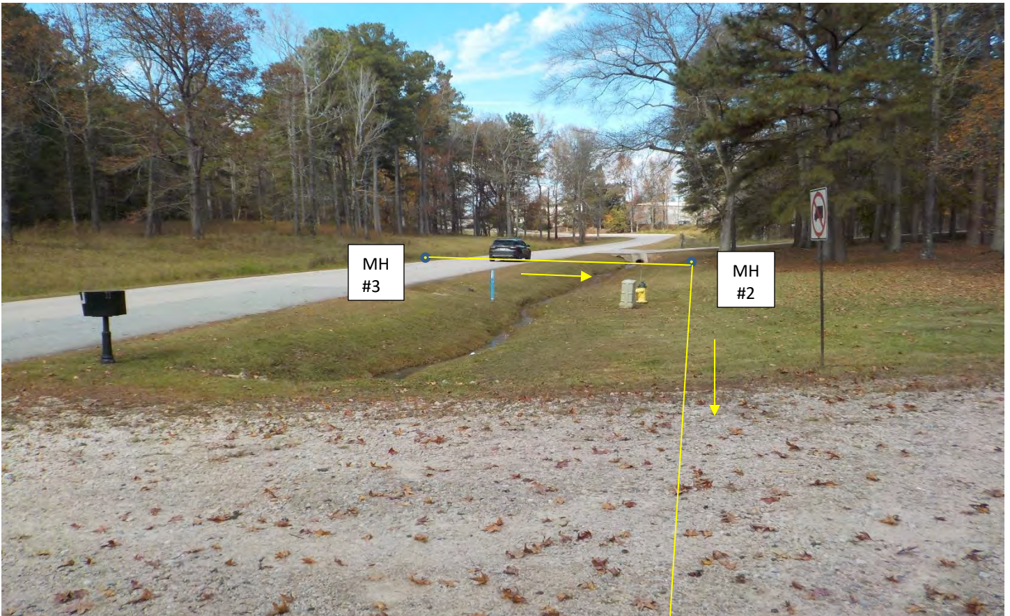
MH #3 to MH #2 to MH #1
