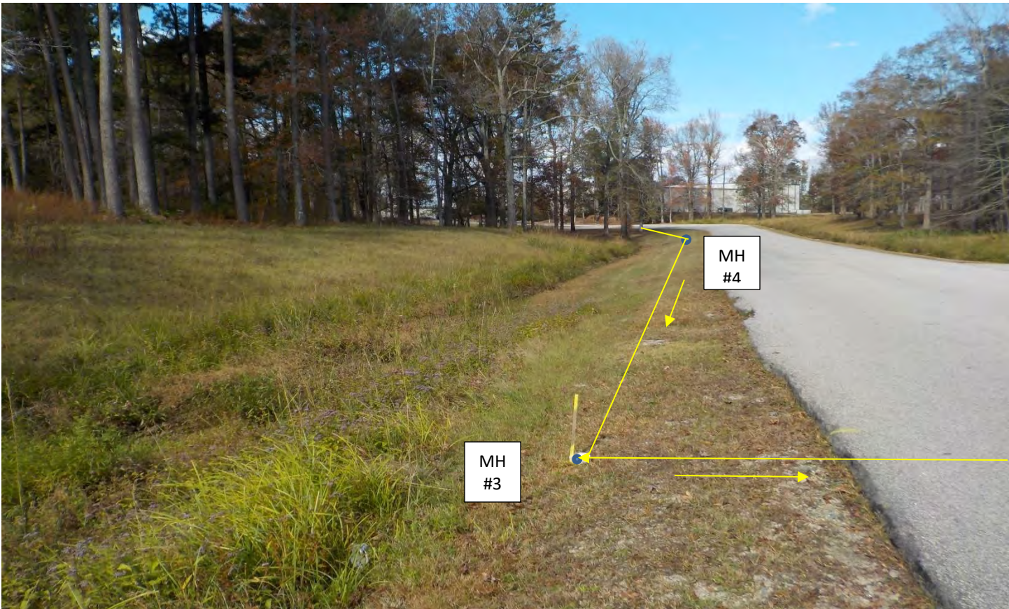
MH #4 to MH #3 to MH #2
