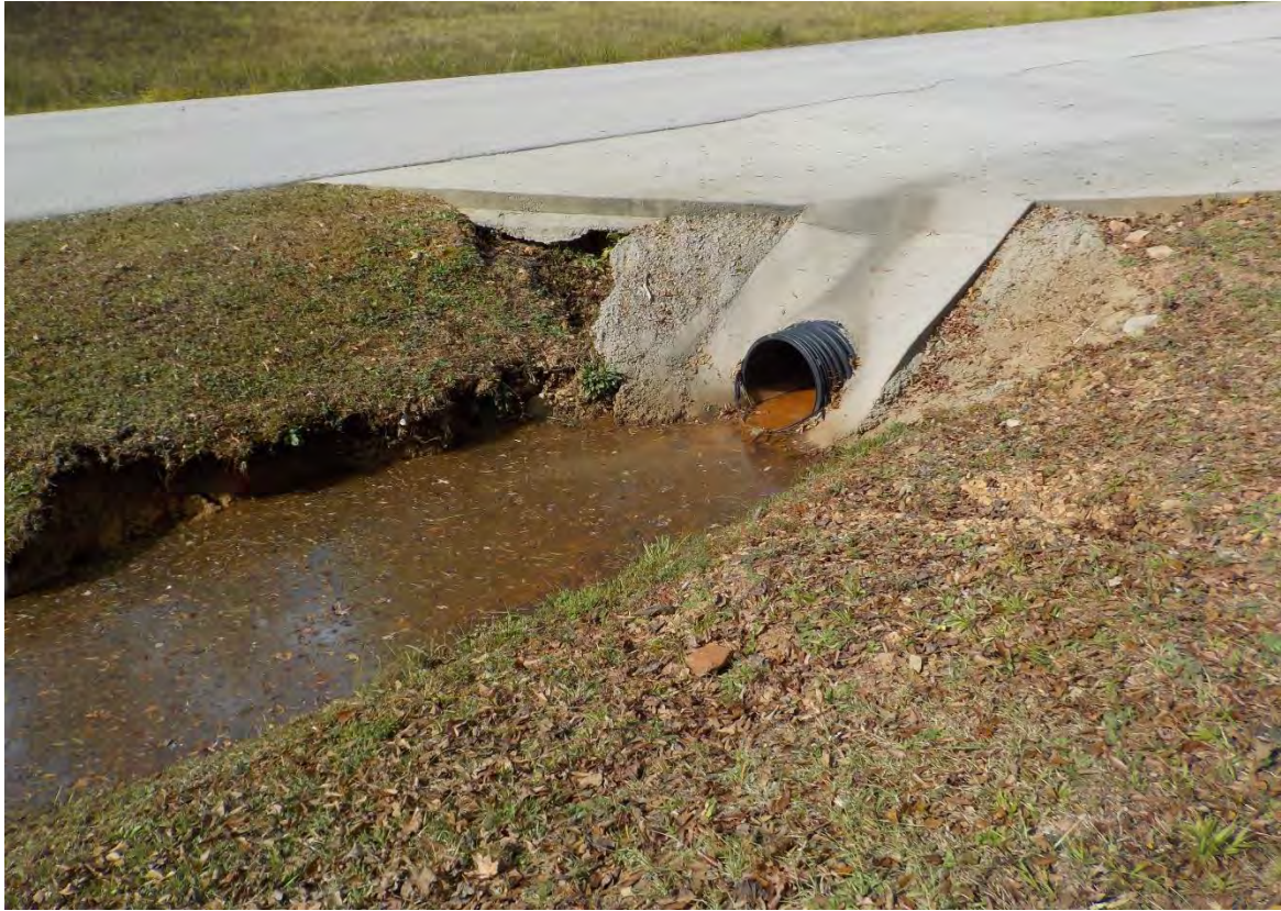
Culvert located just upstream of line MH#2 to MH#3 stream crossing
