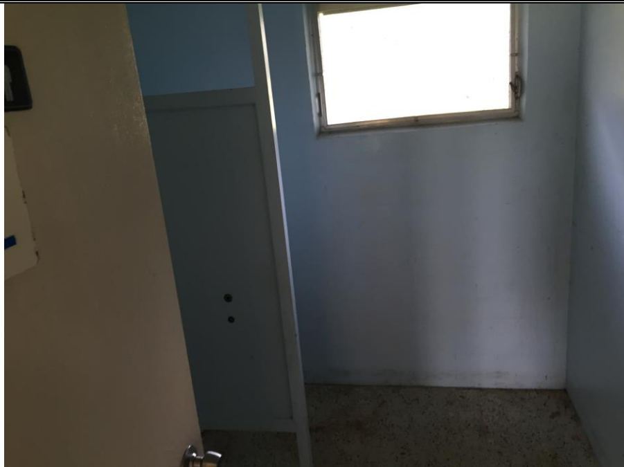
PHOTO # 10: VIEW OF GENERAL INTERIOR CONDITIONS.
