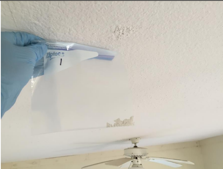
PHOTO # 2: VIEW OF SAMPLED CEILING SURFACING MATERIAL.
