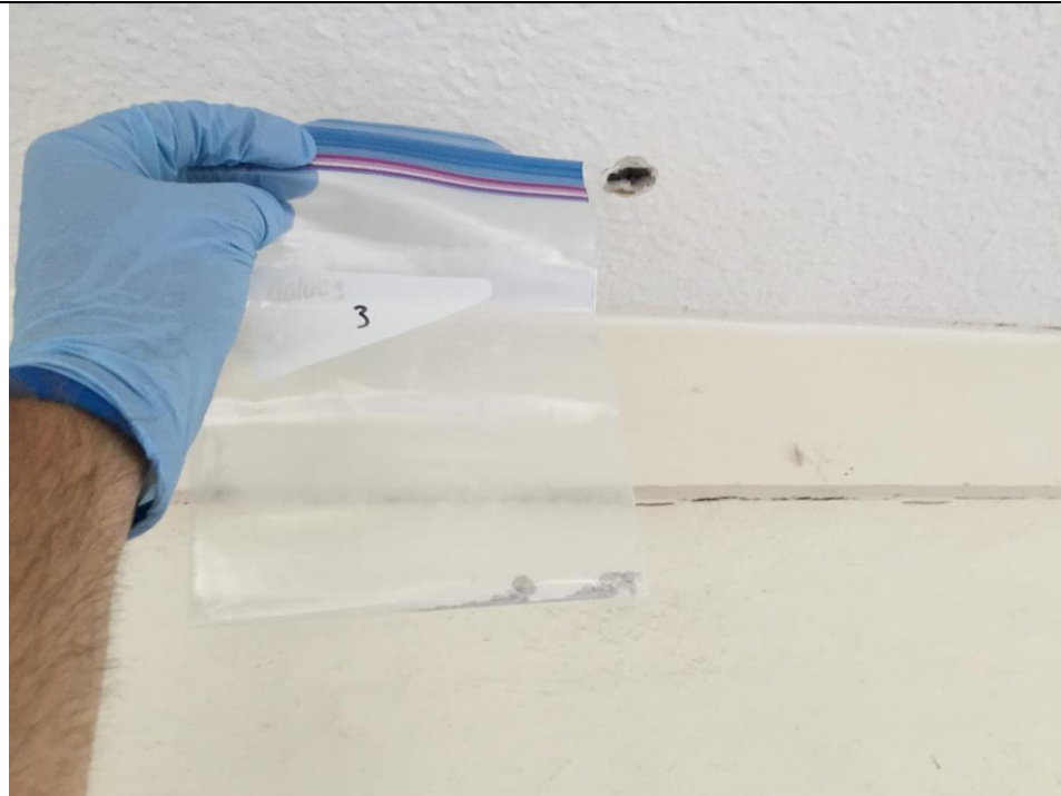
PHOTO # 4: VIEW OF SAMPLED CEILING DRYWALL.
