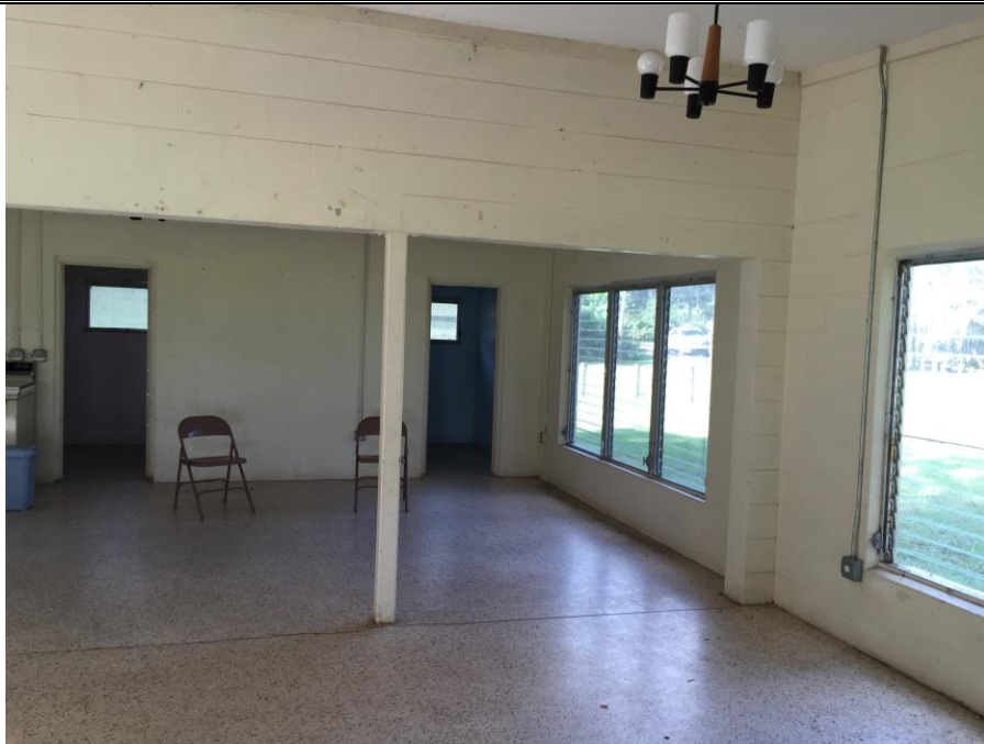
PHOTO # 9: VIEW OF GENERAL INTERIOR CONDITIONS.
