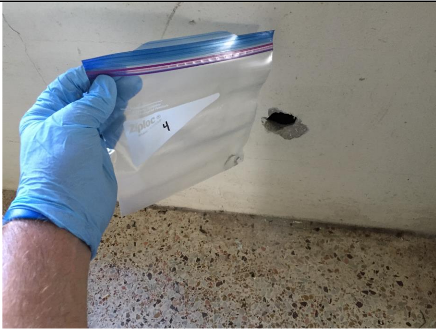
PHOTO # 5: VIEW OF SAMPLED CONCRETE BLOCK.
