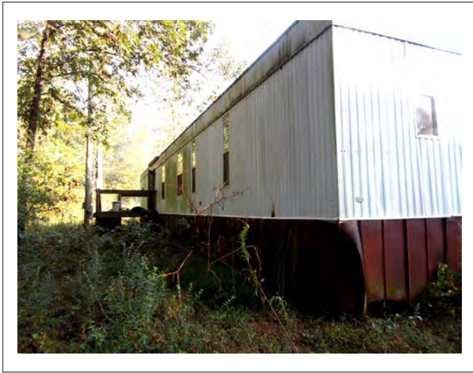
Western side of the mobile home, facing north.
