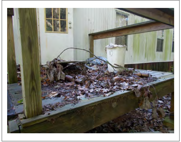
Back porch on western side of the mobile home, facing east.
