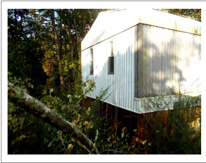
Southern side of the mobile home, facing west.
