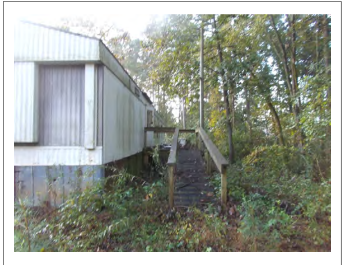
Western side of the mobile home, facing south
