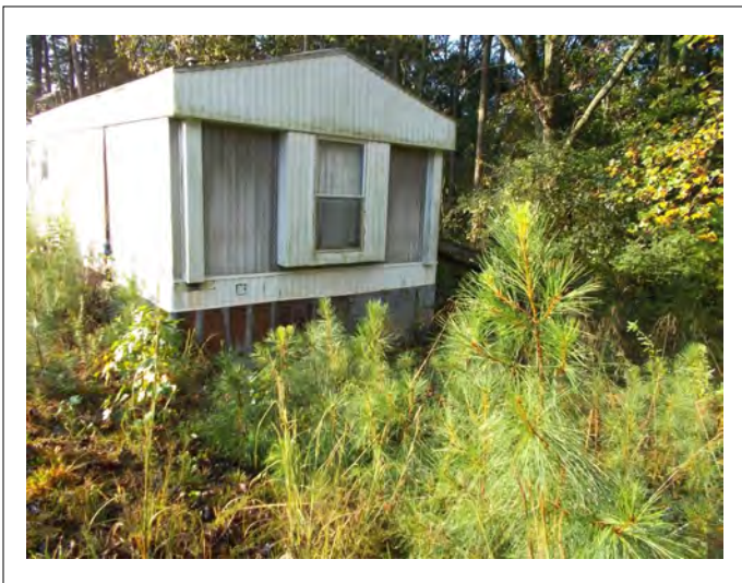
Northern side of the mobile home, facing southwest.
