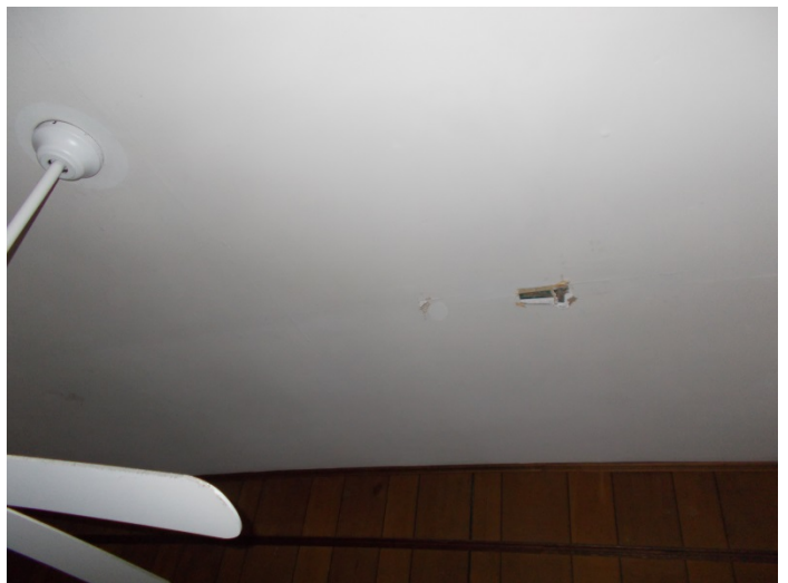
Photo 6 – Drywall with joint compound and tape.
