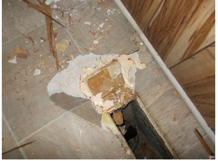
Photo 12 – White floor tile and mastic under wood.
