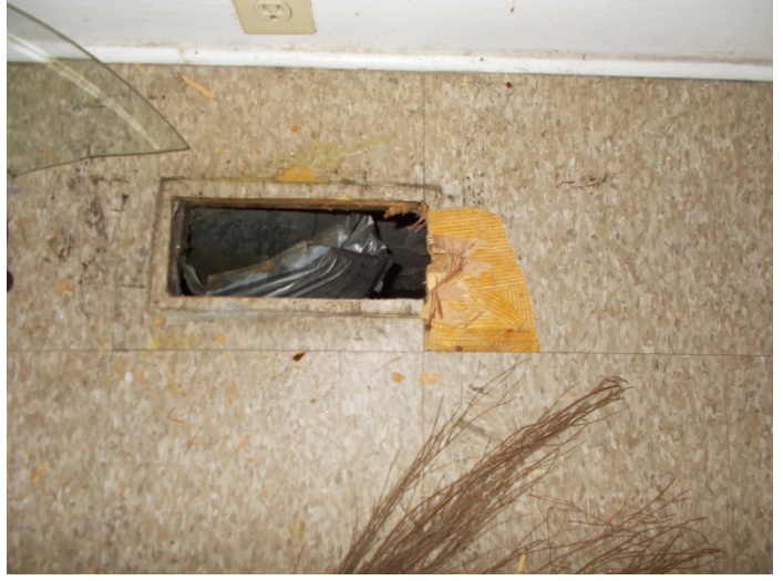
Photo 10 – 12"x12" beige speckled floor tile with mastic.
