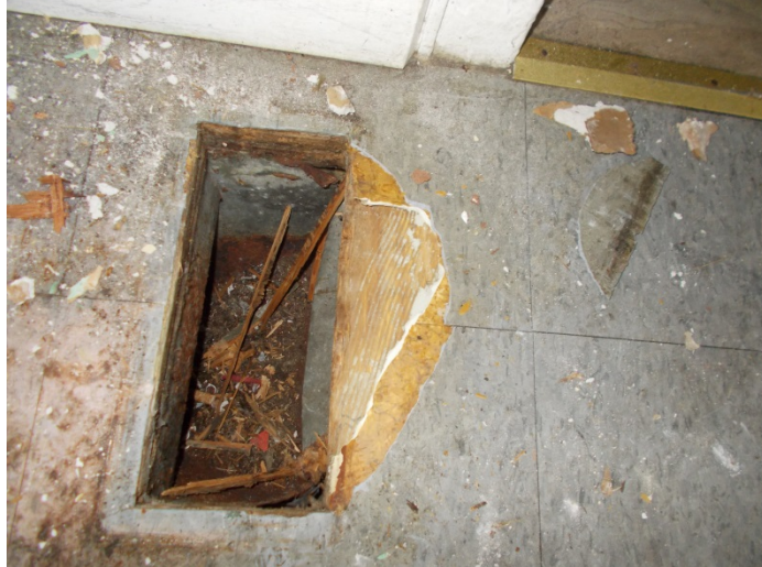
Photo 14 – 12"x12" blue streaked floor tile with mastic over gold / brown pattern vinyl floor with mastic in the laundry room and bathroom.
