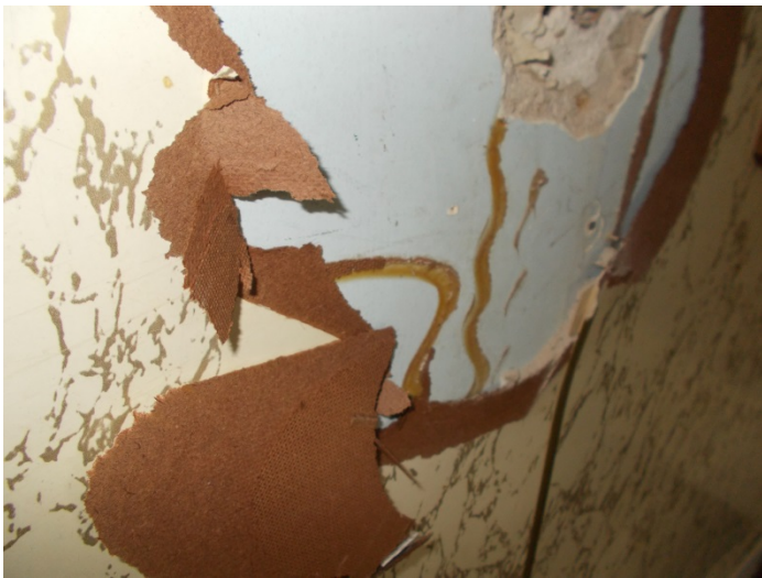
Photo 9 – Wall panel mastic.
