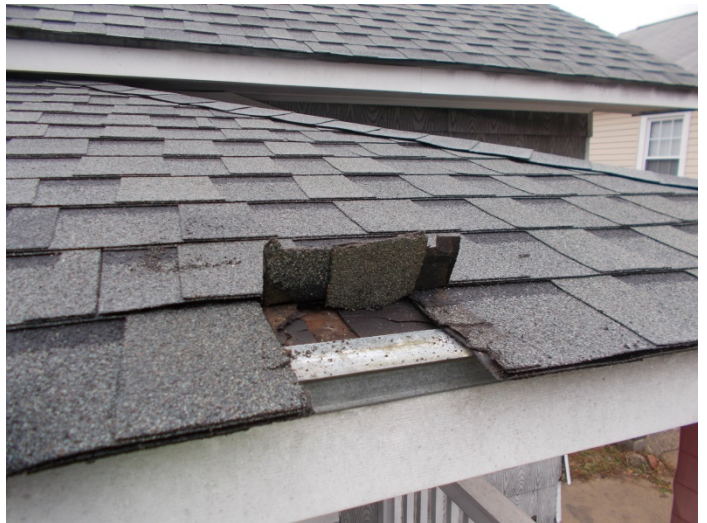
Photo 2 – Roll shingle roof (4) & felt (3).
