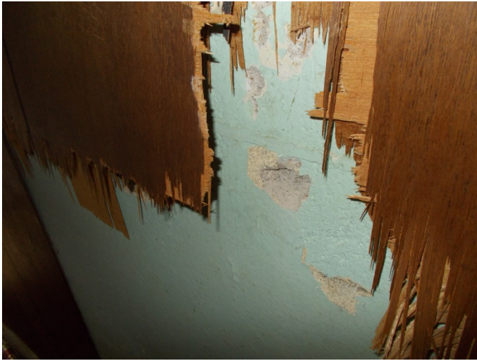
Photo 7 – Plaster with finish.
