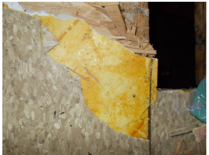
Photo 12 – Yellow pattern vinyl floor with no mastic (3 rd layer).
