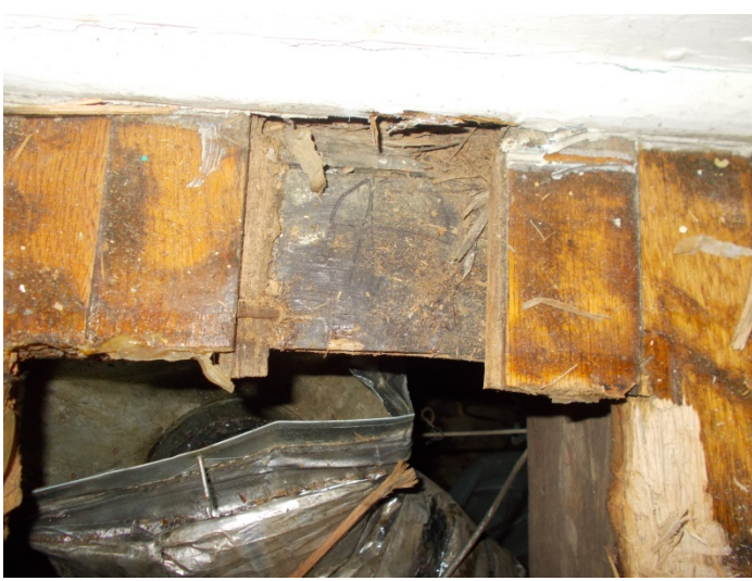
Photo 13 – Flooring paper throughout under wood.
