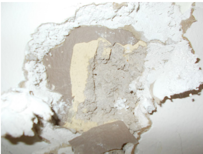
Photo 9 – Plaster with finish.
