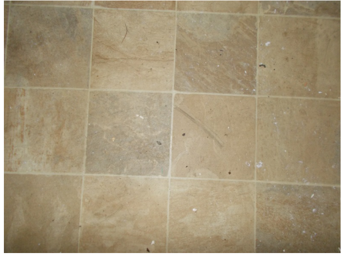
Photo 10 – Slate square pattern vinyl floor with mastic (top layer).
