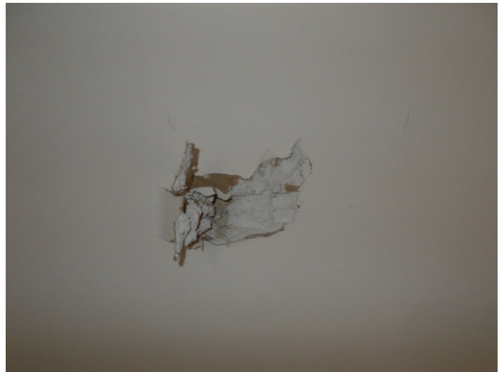
Photo 8 – Drywall with joint compound and tape.
