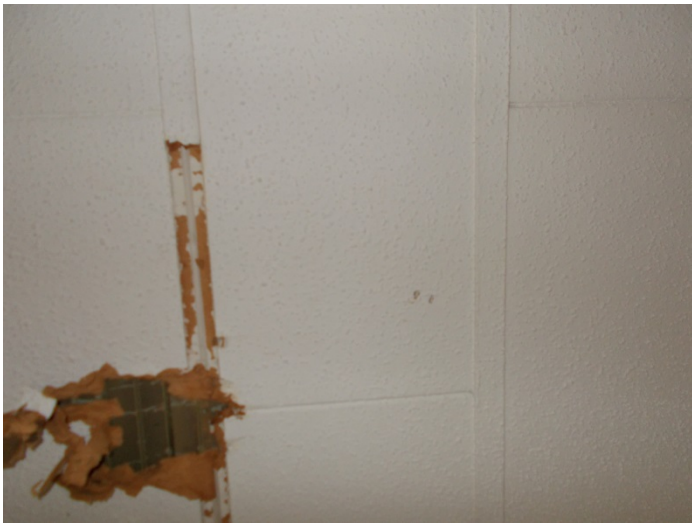
Photo 7 – Ceiling texture over wooden composite ceiling tiles.
