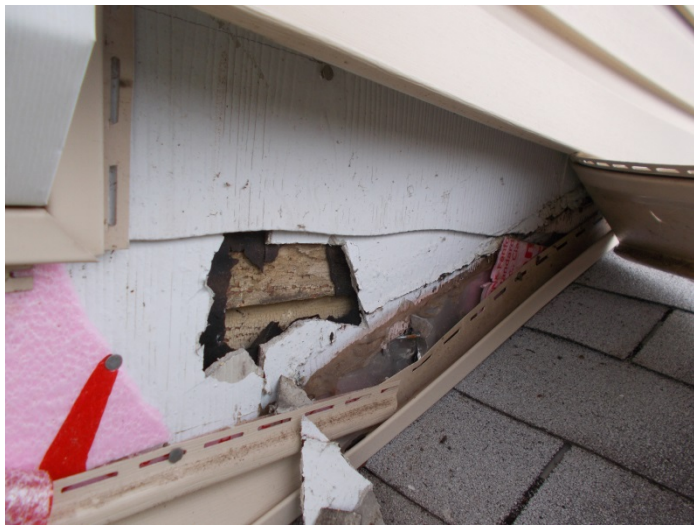
Photo 3 – Cement board siding and felt.
