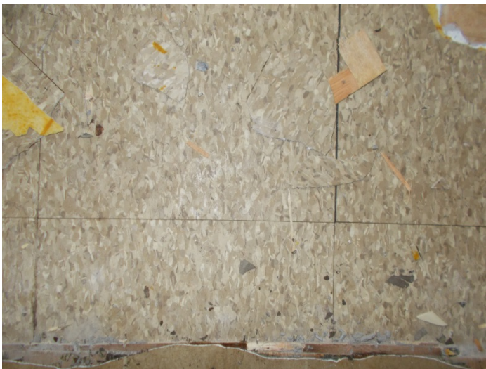
Photo 11 – 12"x12" tan speckled floor tile with mastic (2 nd layer).
