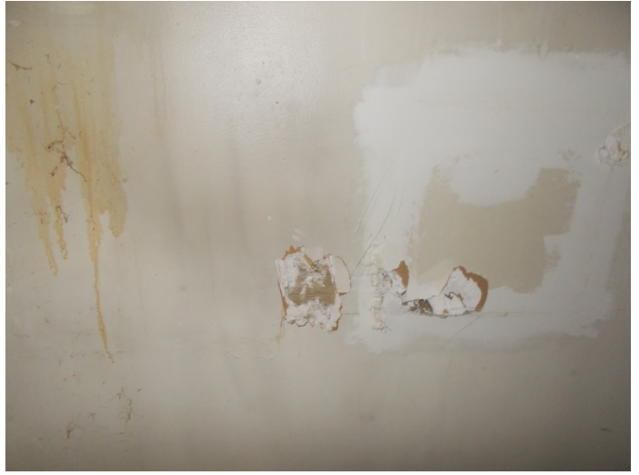
Photo 10 – Drywall with joint compound and tape throughout walls.
