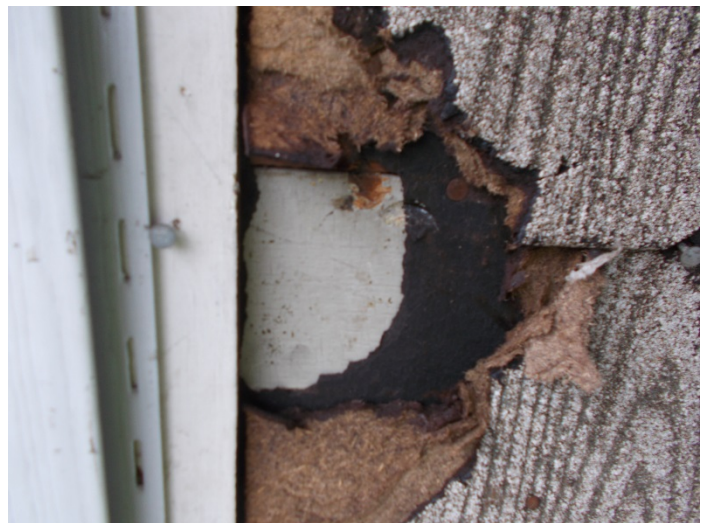
Photo 6 – Siding felt over wood.
