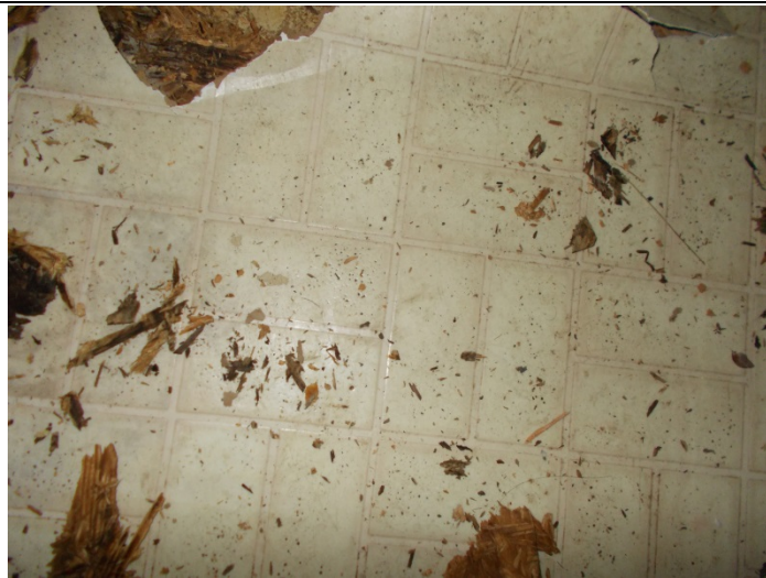
Photo 13 – Tan square pattern vinyl floor with mastic in front right bathroom (top layer).
