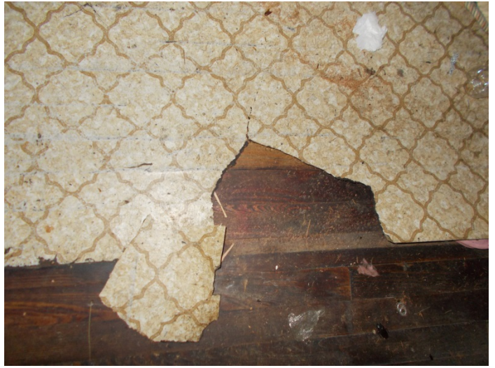
Photo 12 – Brown pattern vinyl floor with no mastic over wood in front right bedroom.
