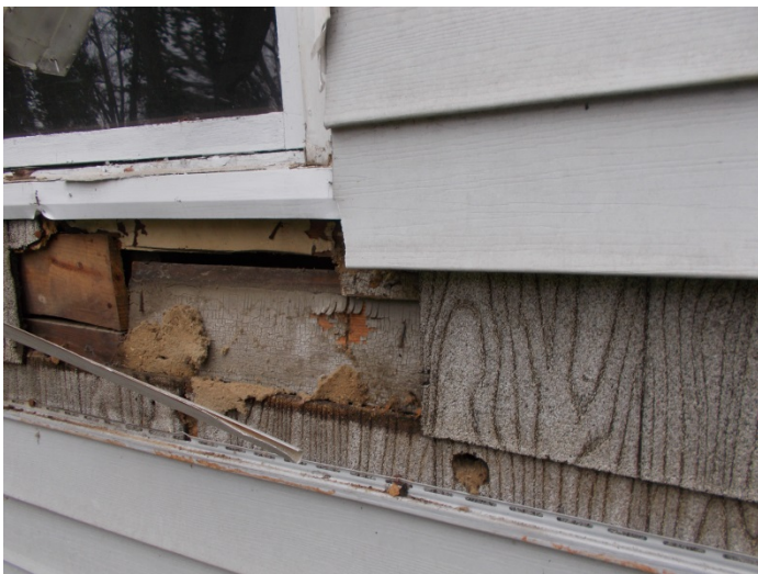
Photo 5 – Shingle siding with felt backing.
