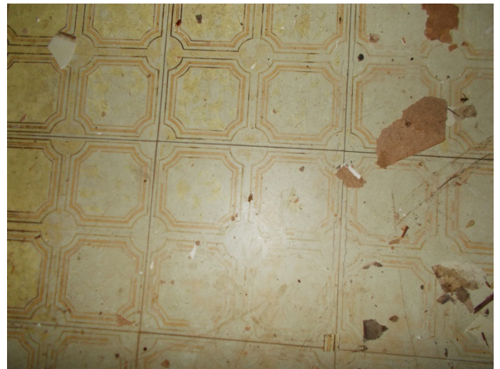
Photo 16 – 12"x12" yellow pattern floor tile with mastic in kitchen (top layer).
