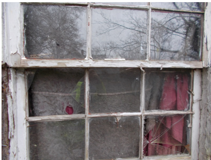
Photo 9 – Window glazing on shed windows.
