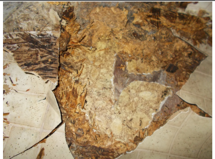
Photo 14 – Yellow pattern vinyl floor with mastic under wood (2 nd layer).
