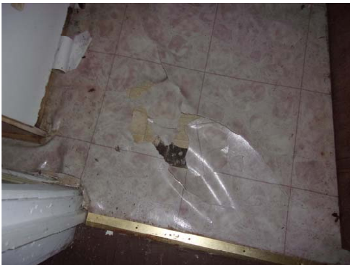
Photo 11 – Grey stone pattern vinyl floor with no mastic in the bathroom (top layer)
