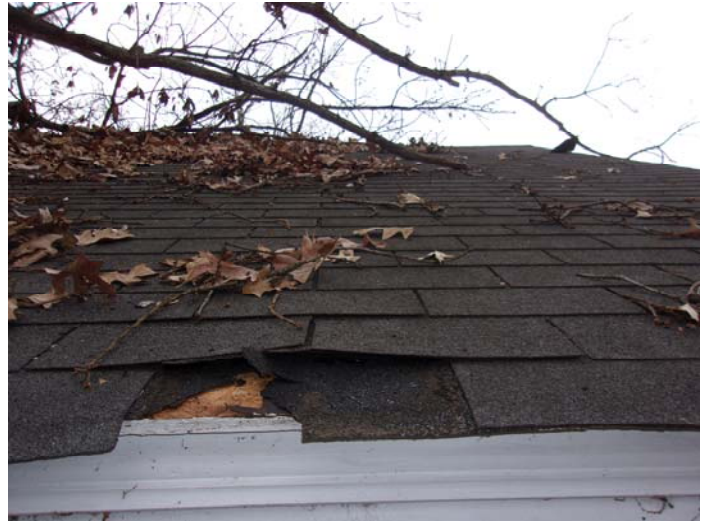
Photo 2 – Roof shingles & felt
