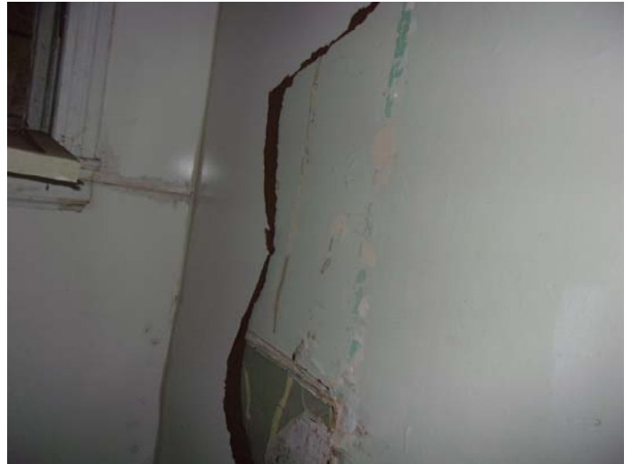
Photo 8 – Drywall with joint compound & tape throughout
