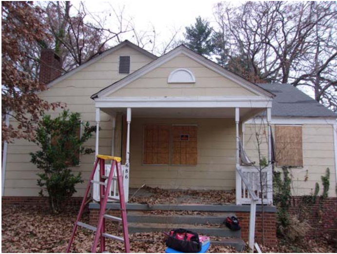
Photo 1 – 686 Saxon Avenue in Spartanburg, South Carolina
