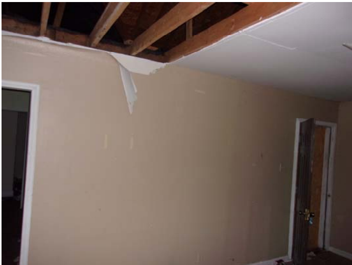
Photo 9 – Drywall with joint compound & tape throughout
