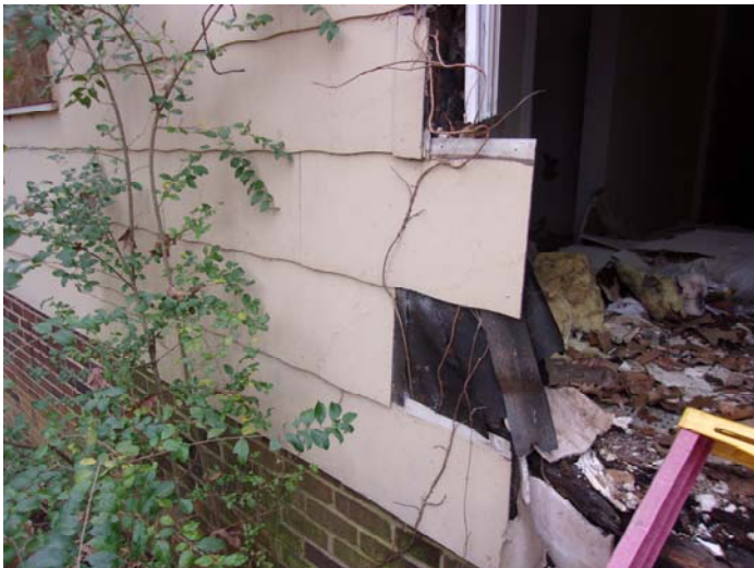
Photo 3 – Cement board siding with felt paper over wood
