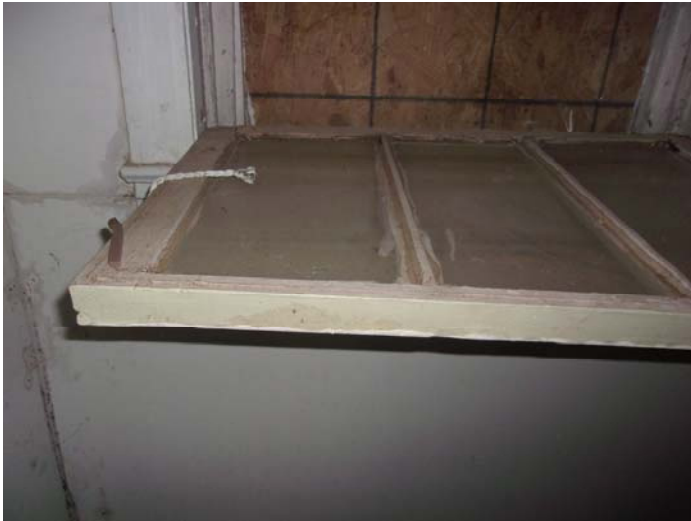
Photo 7 – Window glazing on small wooden bathroom window
