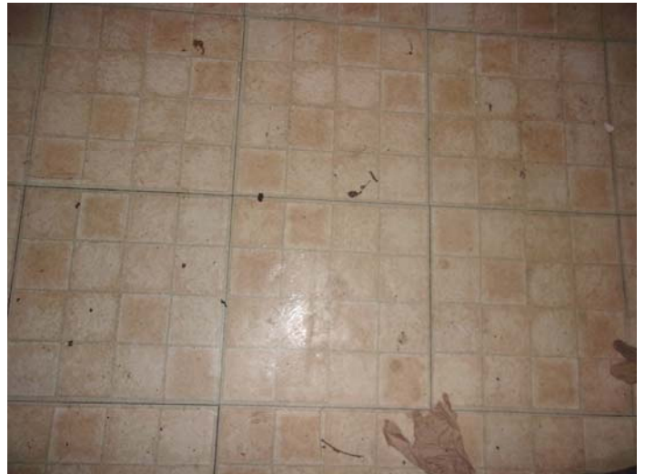
Photo 10 – Tan multi-square pattern self-stick floor tile & tan adhesive in the kitchen (top layer) & bathroom (2 nd layer)
