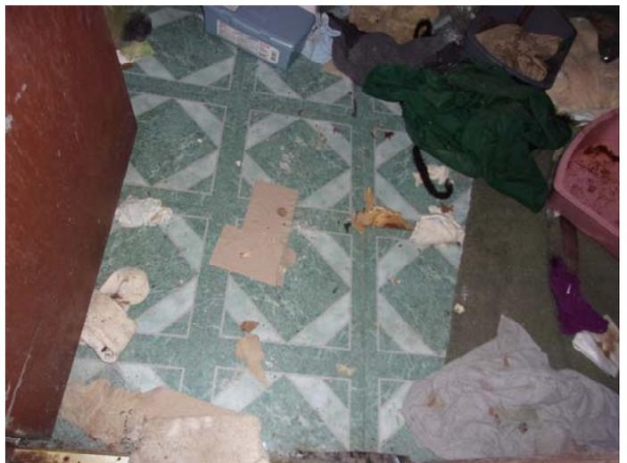
Photo 6 – Brown pattern roll vinyl floor with no mastic over white pattern roll vinyl floor with no mastic in the kitchen & hallway – 2<sup>nd</sup> & 3<sup>rd</sup> layers
