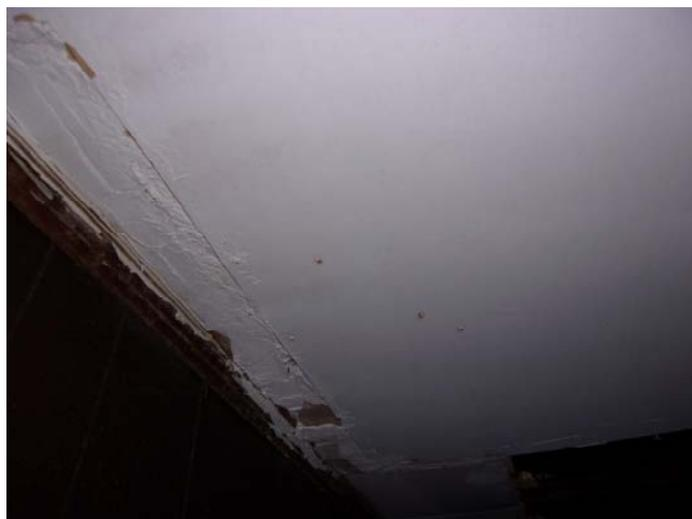
Photo 9 – Joint compound on wooden ceiling in the kitchen & hallway
