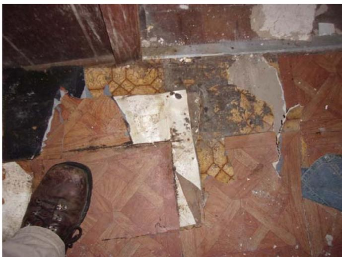
Photo 5 – 12" x 12" wooden pattern self-stick floor tile in the kitchen & hallway – top layer
