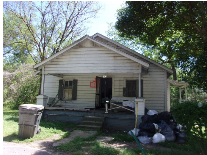
Photo 1 – 583 Carpenter Street in Spartanburg, South Carolina
