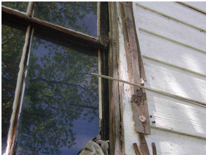
Photo 5 – Wooden window glazing
