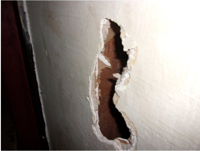
Photo 7 – Plaster with finish over unfinished drywall in the living room & front left bedroom walls
