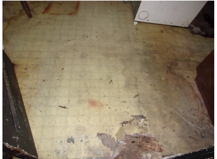
Photo 10 – Tan small square pattern vinyl floor with no mastic in the kitchen
