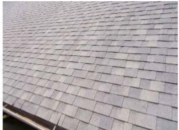
Photo #10 View of the roof of the original main building.
