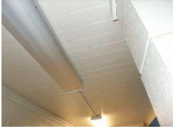
Photo #13 View of the ceiling in the original main building.
