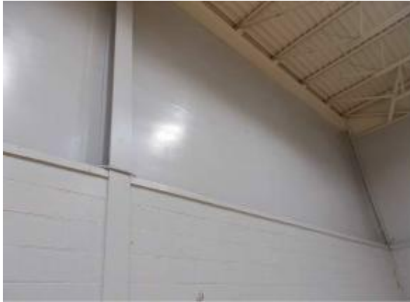
Photo #15 View of walls in the gymnasium.
