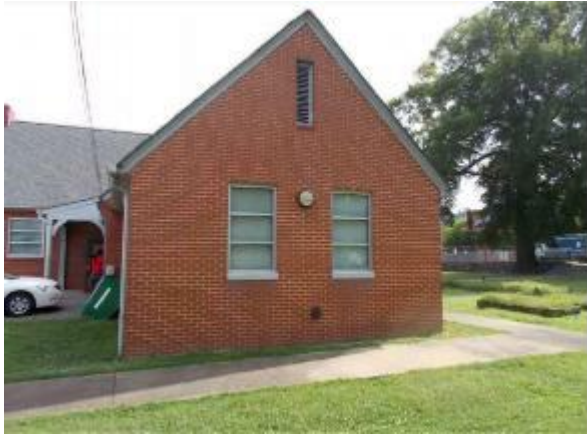
Photo #3 View of the southern exterior facade of the original main building looking northeast from East 37 th Street.
