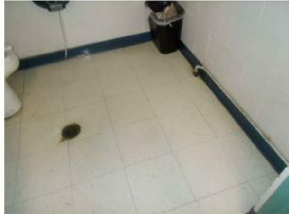
Photo #20 View of the floor tile in the original main building.
