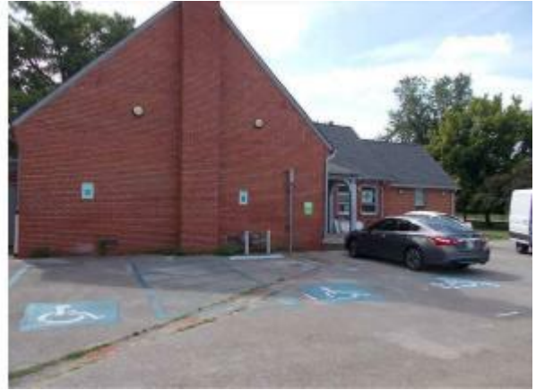
Photo #4 View of the western exterior facade of the original main building looking southeast from the parking lot.
