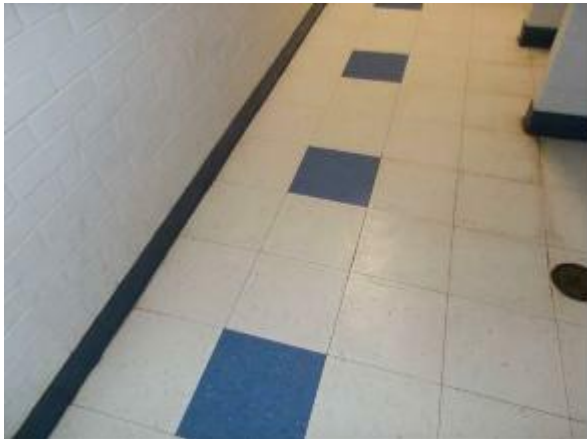
Photo #21 View of the floor tile in the original main building.
