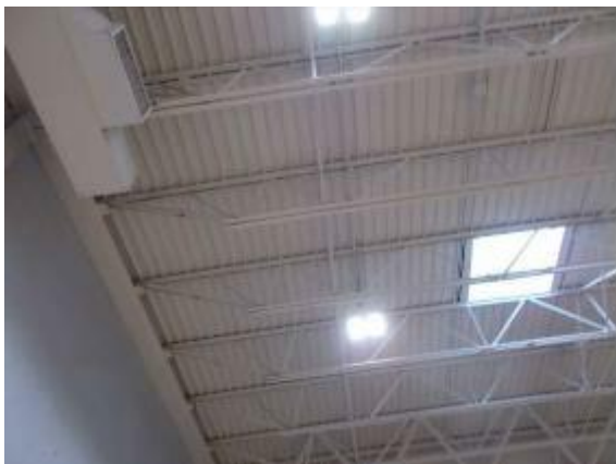
Photo #11 View of ceiling and exposed rafters of the gymnasium building.
