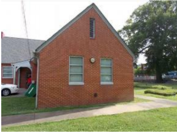
Photo #3 View of the southern exterior facade of the original main building looking northeast from East 37 th Street.
