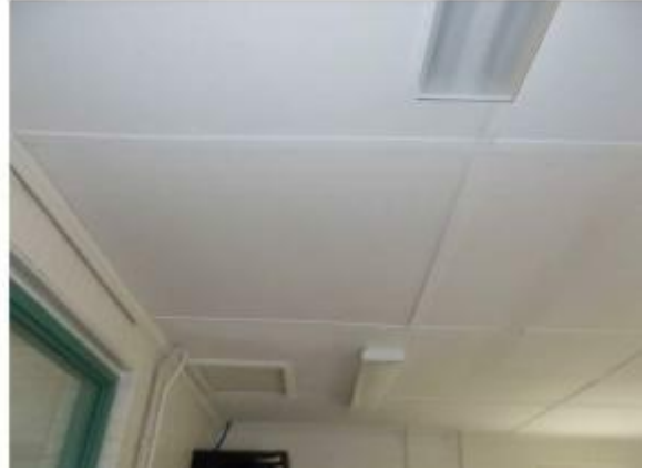
Photo #14 View of the ceiling in the original main building.
