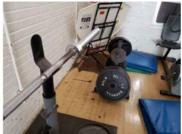
Photo #18 View of floor and walls in the original main building.
