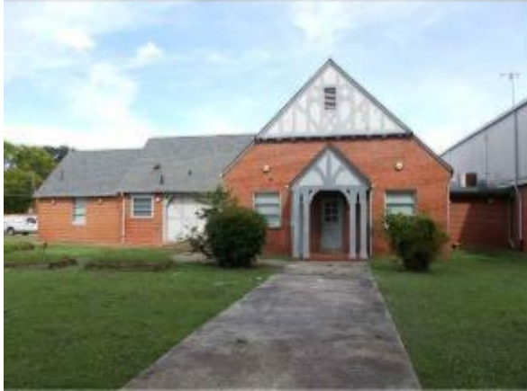
Photo #1 View of the eastern exterior facade of the original main building looking northwest from Dodds Avenue.
