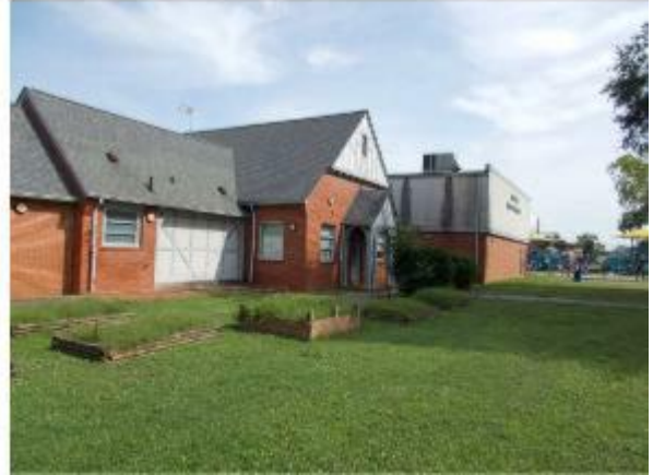
Photo #2 View of the original main building looking north.
