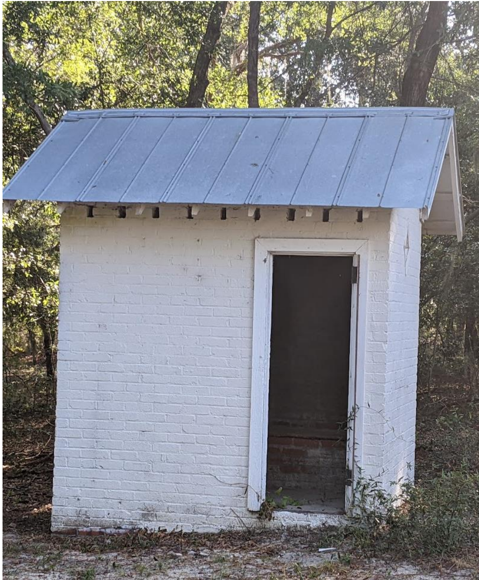
Exterior Outhouse #1-Install New Door.
