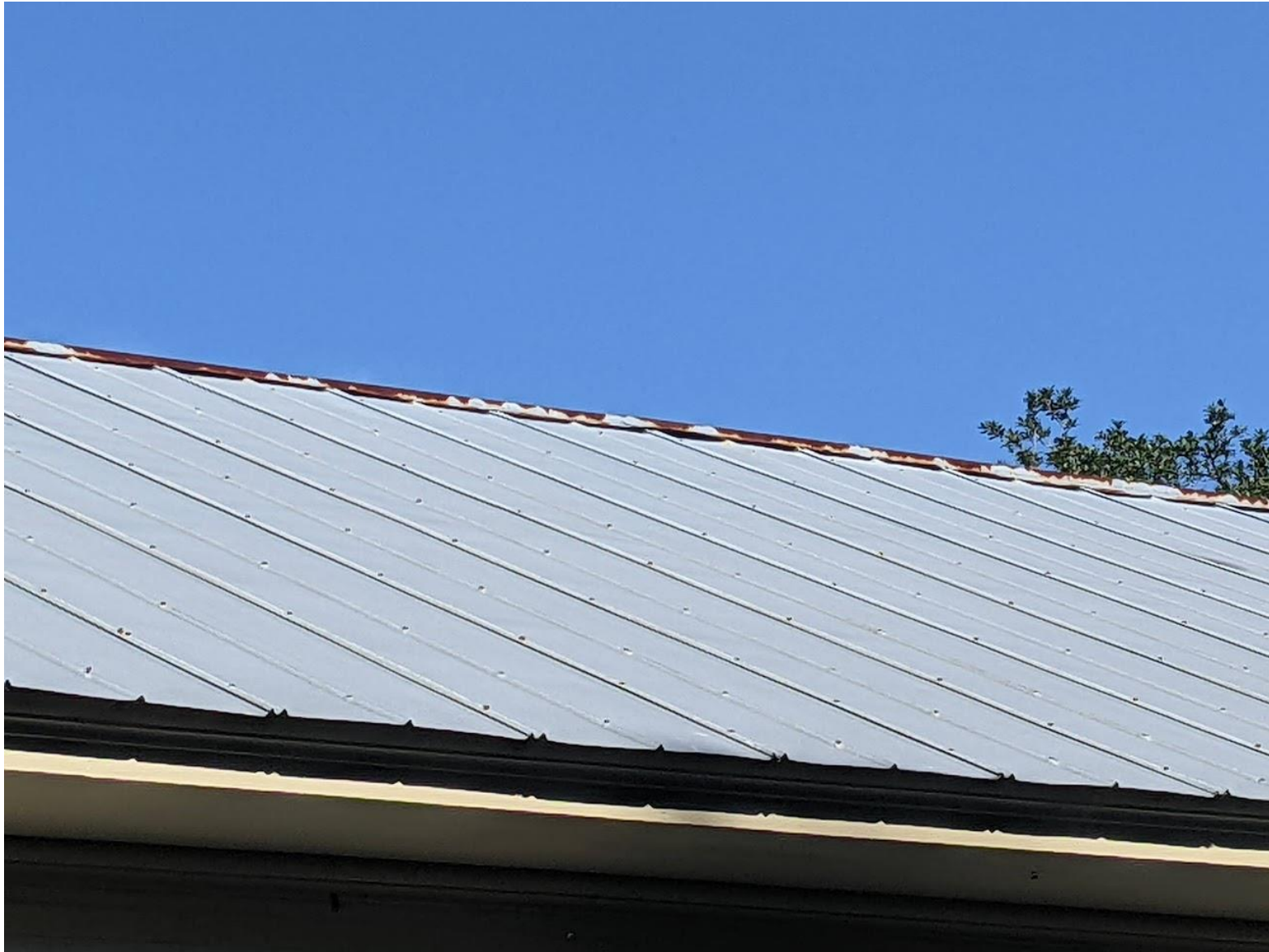
View of roof from the right side of school house-Picture 2
