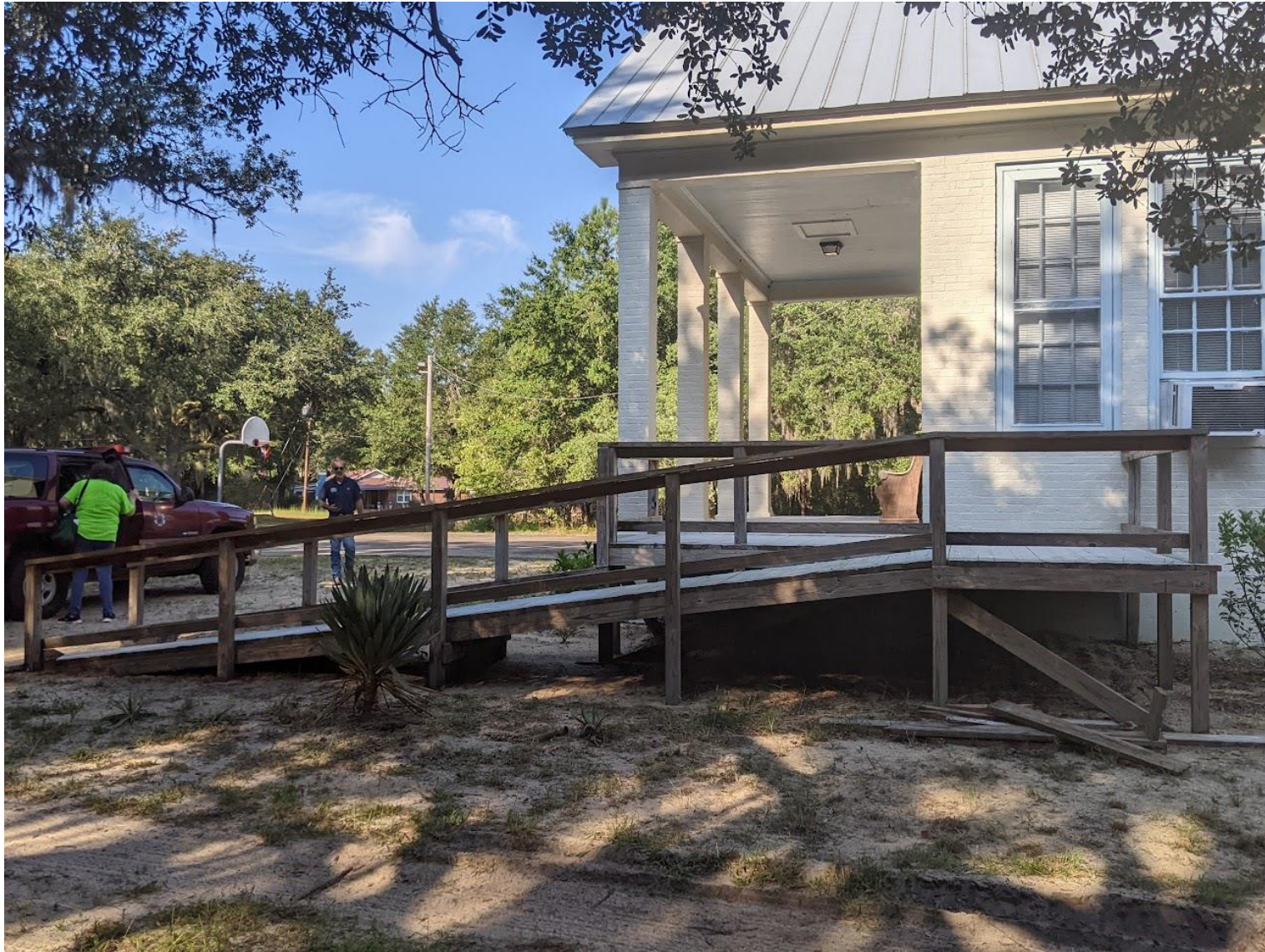
Exterior ADA Ramp to be demoed and rebuilt.
