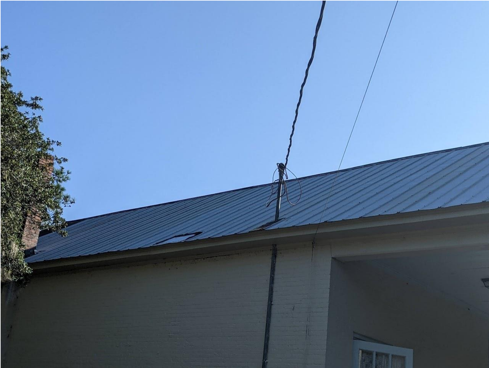
View of roof from the left side of school house-Picture 1
