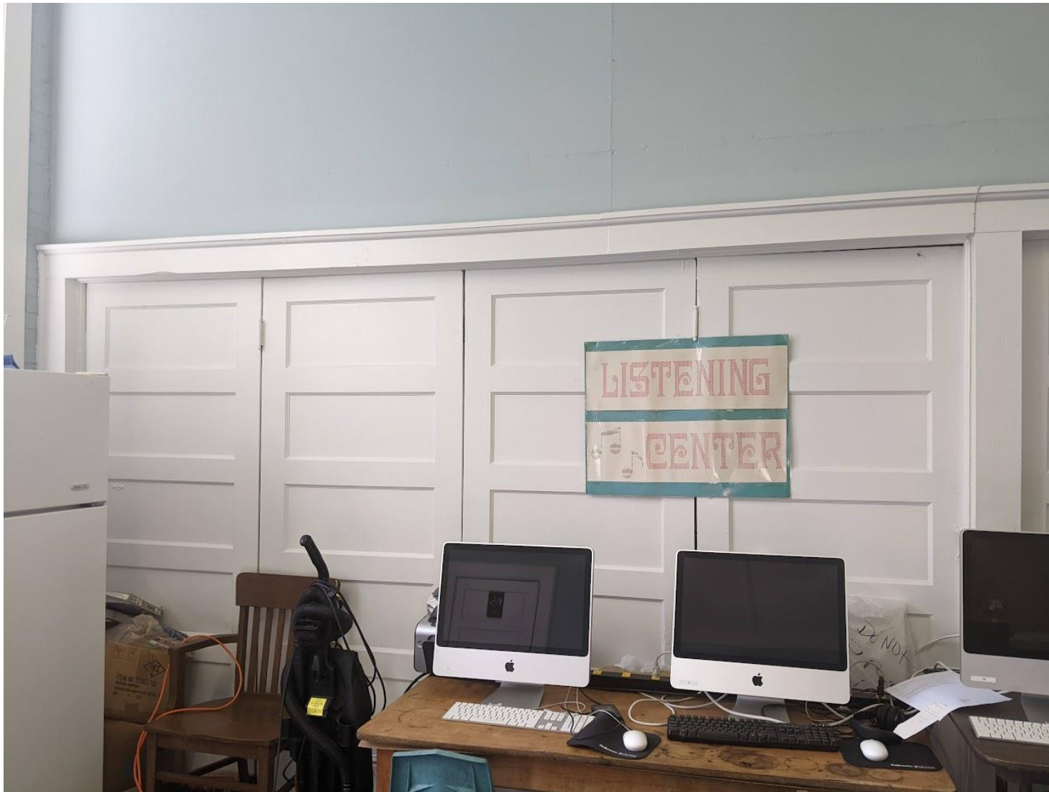
Interior folding doors to make operational – Picture 1
