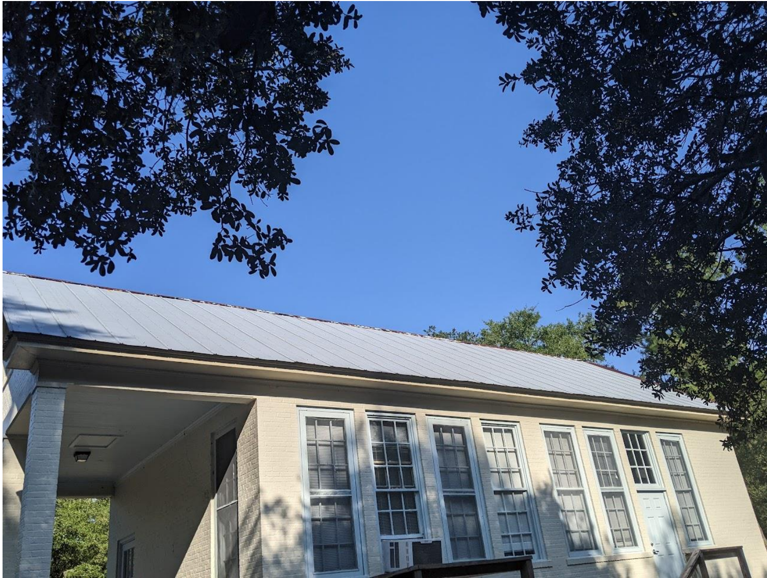
View of roof from the right side of school house-Picture 1
