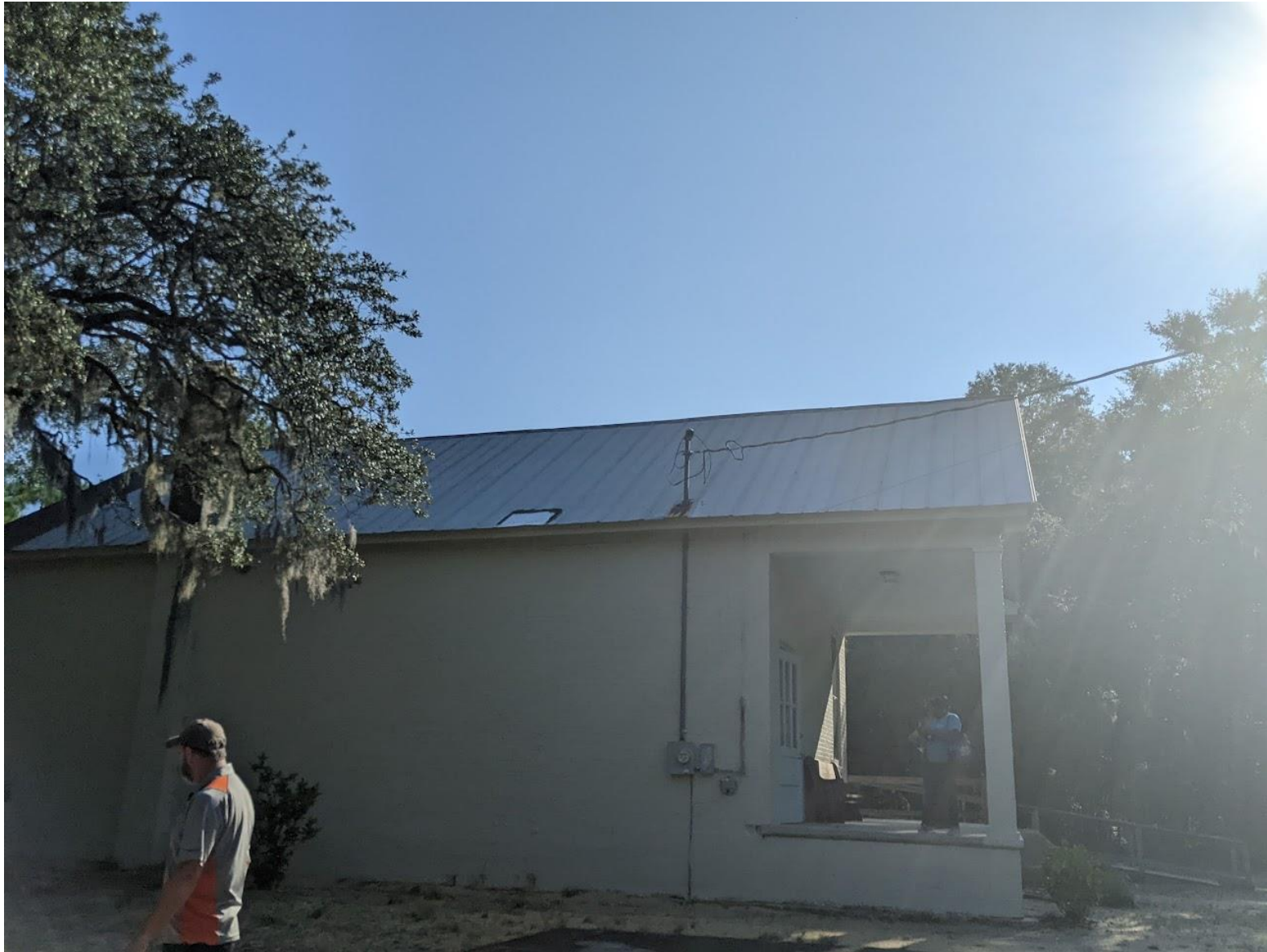
View of roof from the left side of school house-Picture 2
