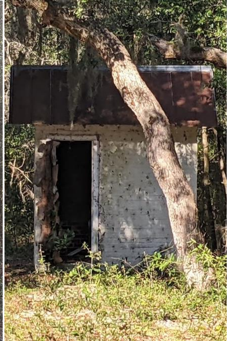
Exterior Outhouse #2-Install New Door.
