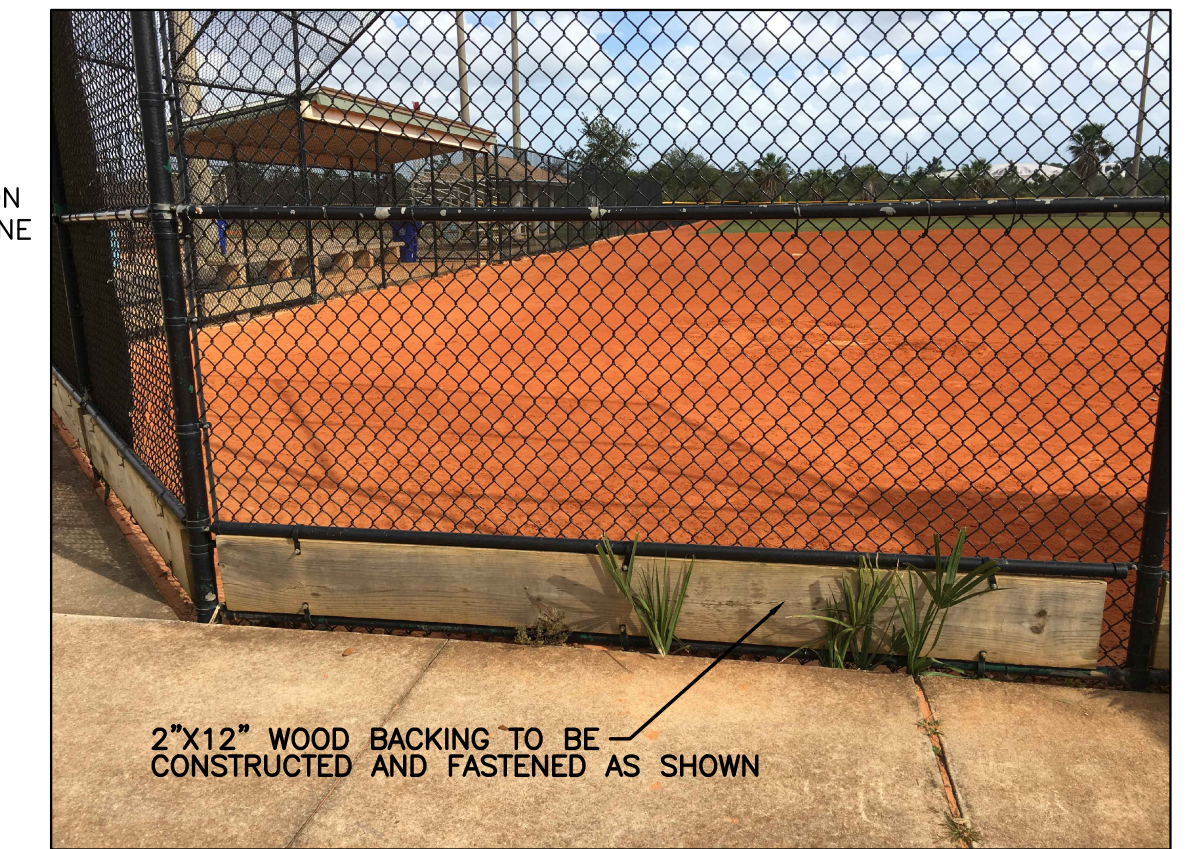
BACKSTOP WOODEN FENCE BACKING
