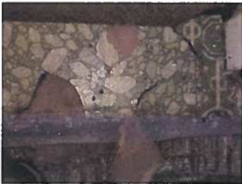
HOMOGENEOUS AREA 23 VINYL SHEET FLOORING (GREEN ROCKS)
