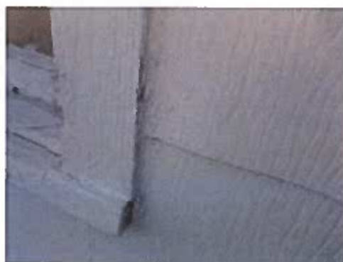
HOMOGENEOUS AREA 04 EXTERIOR CAULK
