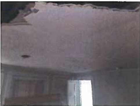
HOMOGENEOUS AREA 11 CEILING TEXTURE (TEXTURE)
