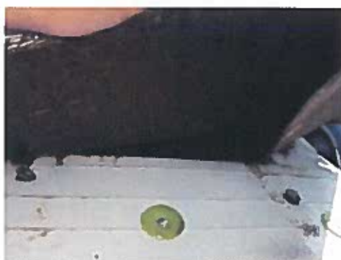
HOMOGENEOUS AREA 06 ROOF FELT
