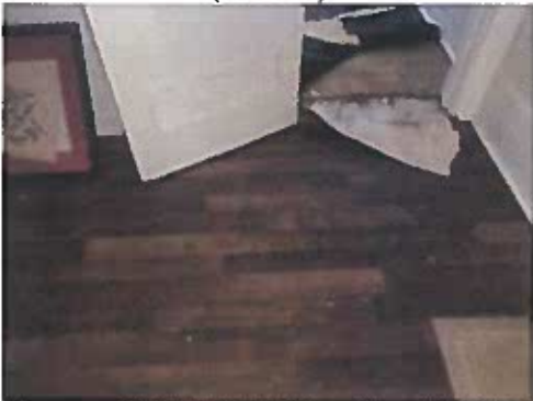
HOMOGENEOUS AREA 23 VINYL SHEET FLOORING (DARK WOOD)
