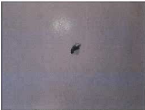
HOMOGENEOUS AREA 09 DRYWALL
