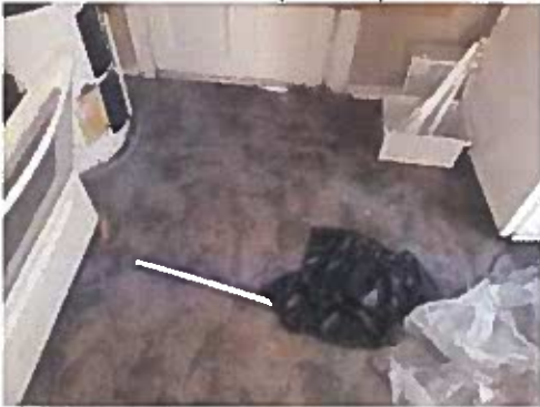
HOMOGENEOUS AREA 21 VINYL SHEET FLOORING (STONE)
