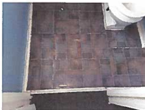
HOMOGENEOUS AREA 10 12" SELF-STICK FLOOR TILE (SLATE)
