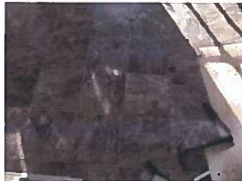
HOMOGENEOUS AREA 16 VINYL SHEET FLOORING (12" SLATE SQUARES)
