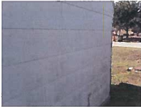
HOMOGENEOUS AREA 01 TRANSITE SIDING
