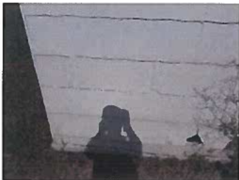
HOMOGENEOUS AREA 01 TRANSITE PANEL
