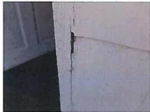
HOMOGENEOUS AREA 04 EXTERIOR CAULK
