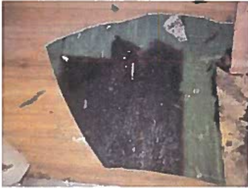
HOMOGENEOUS AREAS 19, 20 9" FLOOR TILE (GREEN) MASTIC (BLACK)
