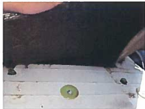
HOMOGENEOUS AREA 06 ROOF FELT
