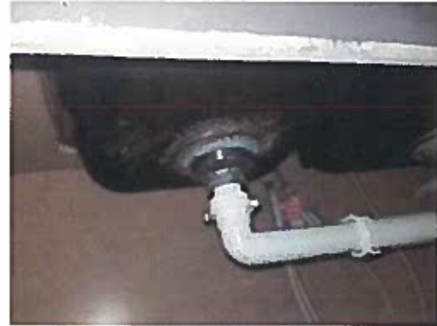
HOMOGENEOUS AREA 08 SINK COATING (BLACK)
