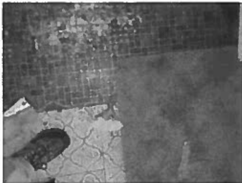
HOMOGENEOUS AREA 16 VINYL SHEET FLOORING (RED BRICK)
