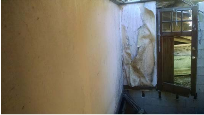
Photo 7 – Drywall with joint compound and tape throughout the ceilings and a quarter of the walls.
