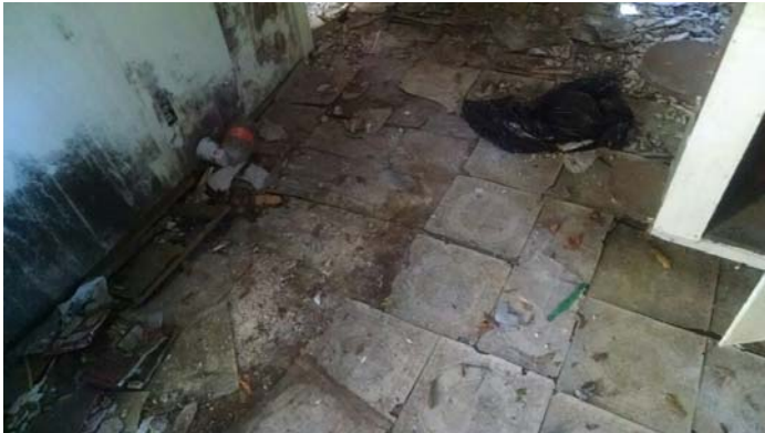
Photo 9 – 12"x12" beige flooring over grey roll vinyl with mastic in the kitchen.
