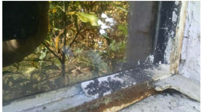
Photo 4 – Exterior windows with glazing.
