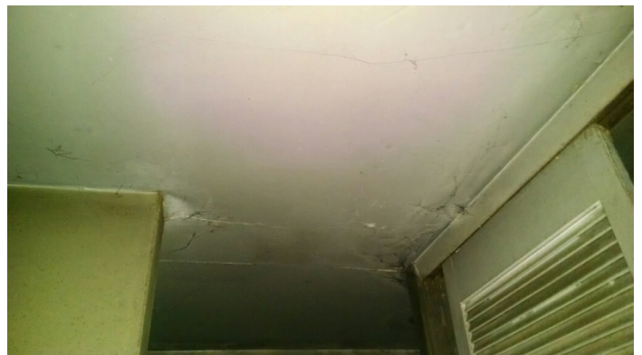
Photo 5 – Drywall with joint compound.
