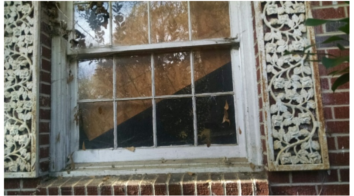
Photo 2 – Windows with glazing.
