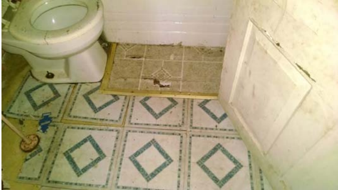
Photo 7 – Bathroom flooring yellow roll vinyl, tan roll vinyl, white 12"x12" self-stick vinyl flooring.
