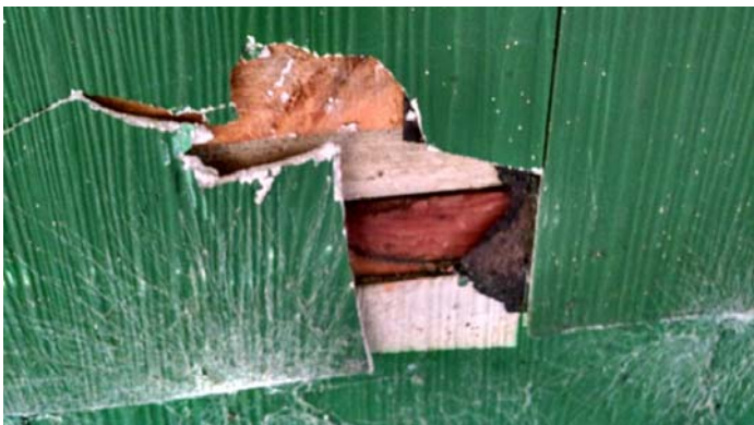
Photo 11 – Cement board siding with felt paper.
