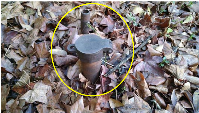
Photo 5 – Underground fuel-tank stub-out in side yard.
