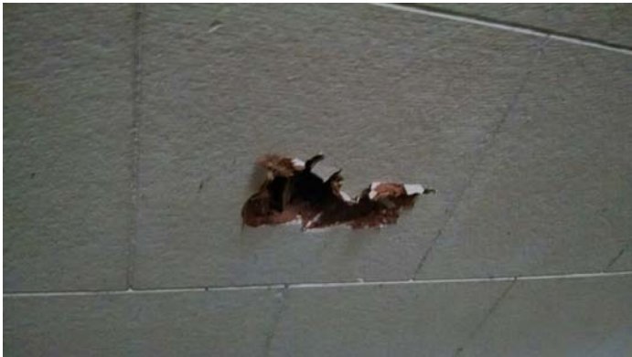
Photo 9 – 1'x1' ceiling tiles.
