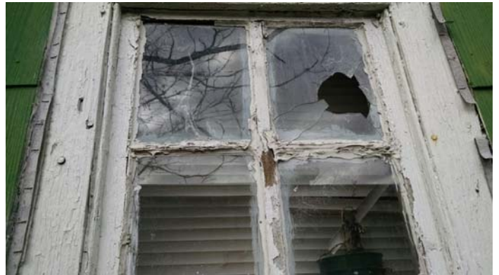
Photo 4 – Window caulk and glazing on exterior windows.
