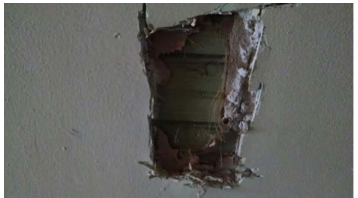
Photo 6 – Drywall walls with joint compound.
