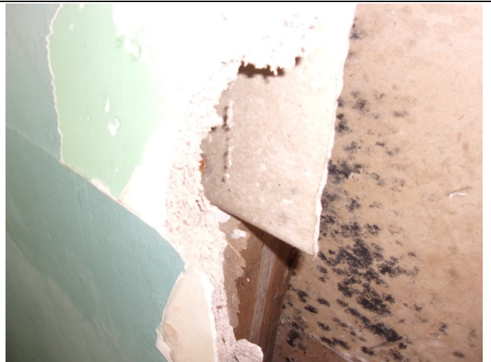
Photo 8 – Plaster with finish over unfinished drywall throughout.
