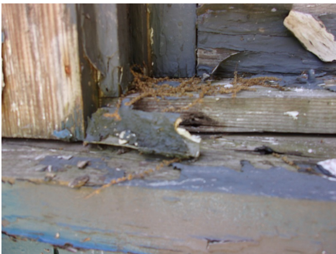
Photo 5 – Wooden window glazing.
