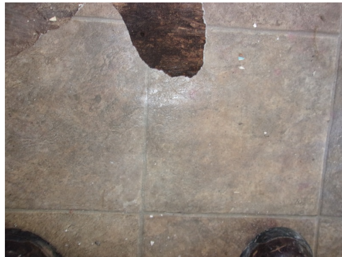
Photo 9 – Brown large square pattern vinyl floor with no mastic in the kitchen.
