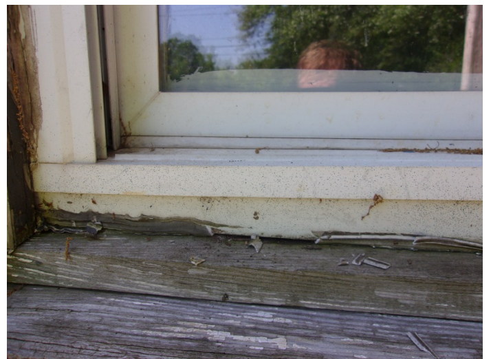
Photo 6 – Vinyl window caulk.
