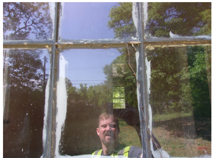
Photo 4 – Wooden window caulk.
