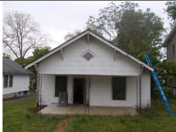
Photo 1 – 735 Fulton Avenue in Spartanburg, South Carolina.
