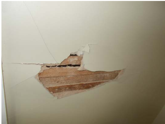
Photo 9 – Plaster with finish throughout interior.
