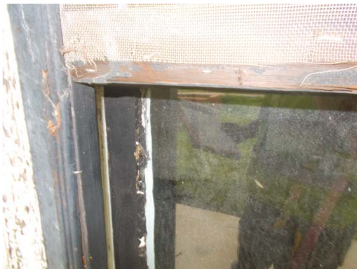
Photo 5 – Glazing on wooden windows.
