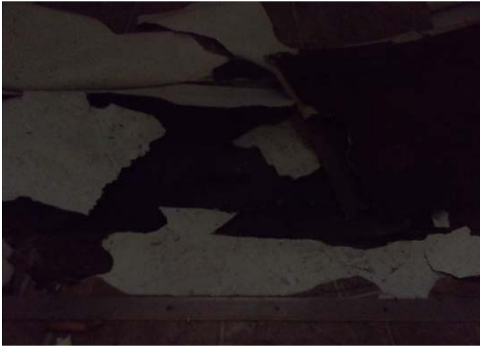
Photo 13 – White pattern vinyl floor with no mastic over dark vinyl floor with no mastic in pantry (2 nd and 3 rd layers).
