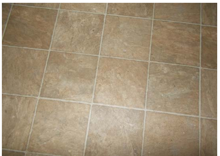
Photo 10 – Dark tan square pattern vinyl floor with no mastic in kitchen and pantry (top layer).
