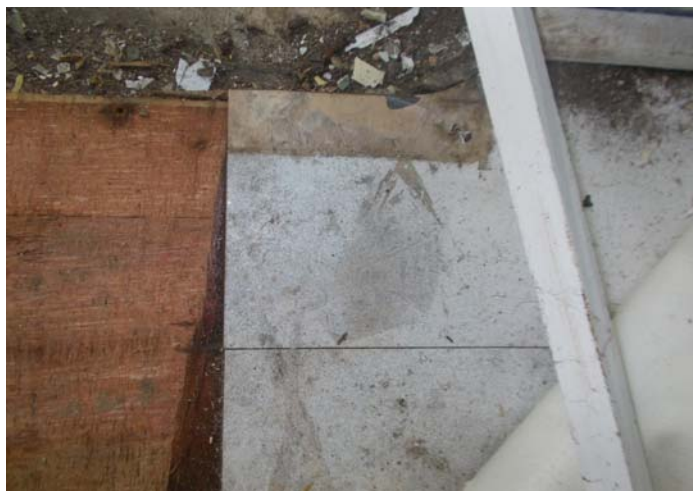
Photo 11 – 12"x12" grey floor tile in kitchen (2 nd layer).
