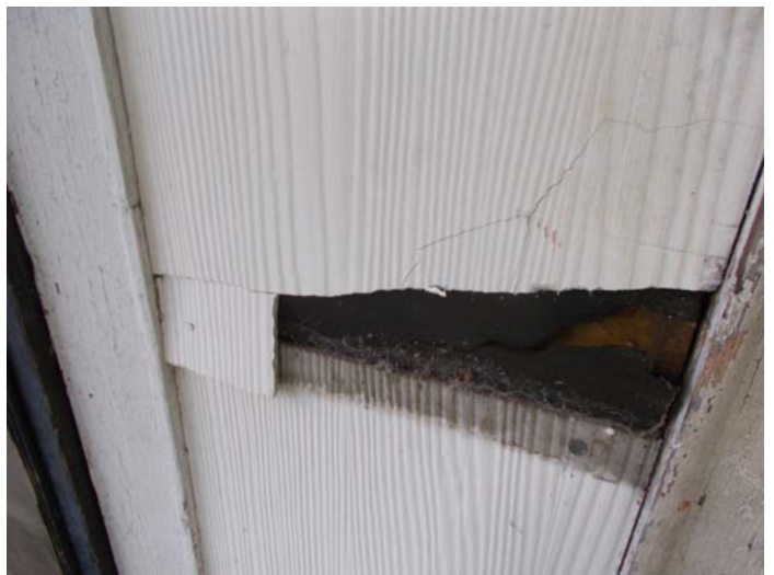
Photo 4 – Cement board siding with felt beneath.
