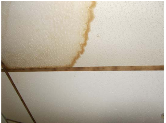
Photo 8 – 2'x4' pinhole ceiling tiles in middle left room.
