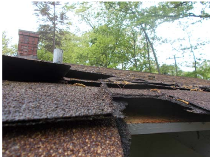
Photo 2 – Roofing material (4 layers) and felt (1 layer).
