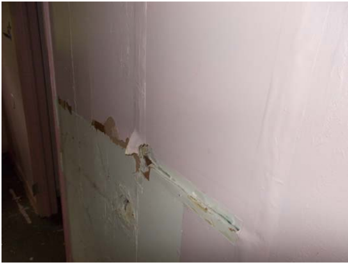
Photo 7 – Drywall with tape and coating throughout interior.
