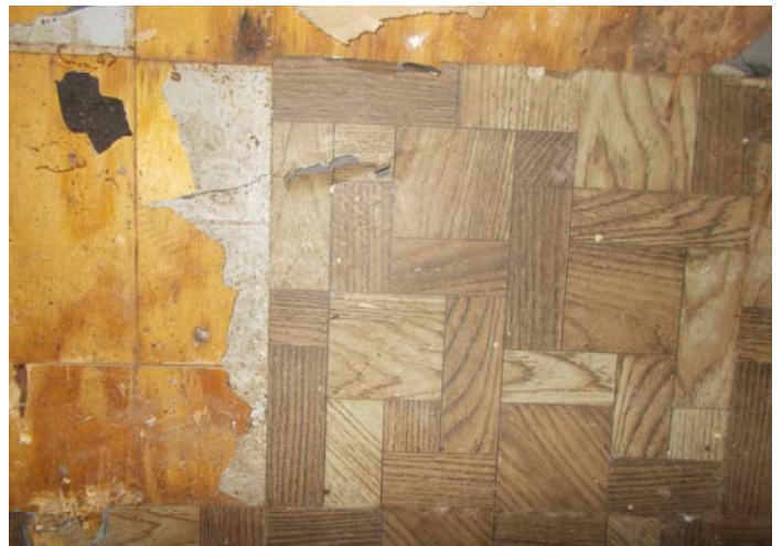
Photo 10 – 12"x12" wood pattern self-stick floor tile and 12"x12" grey self-stick floor tile.
