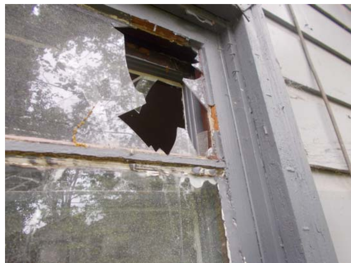
Photo 5 – Caulk and glazing on exterior wooden window.
