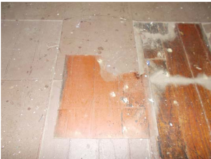
Photo 9 – 12"x12" dark orange floor tile with mastic in the right rear bedroom.
