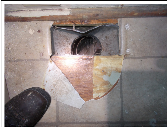
Photo 13 – Beige square pattern vinyl floor with no mastic over wooden pattern vinyl floor with mastic.
