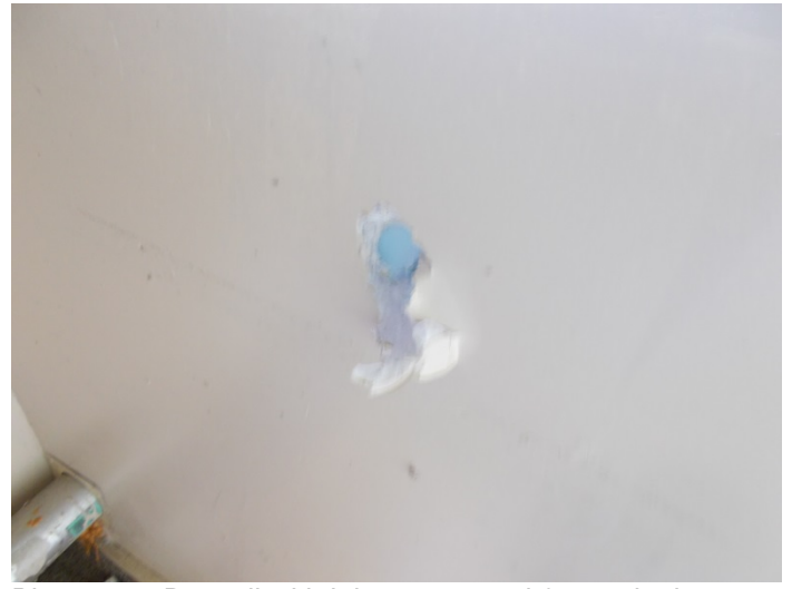
Photo 10 – Drywall with joint compound & tape in the rear entry & bathroom.
