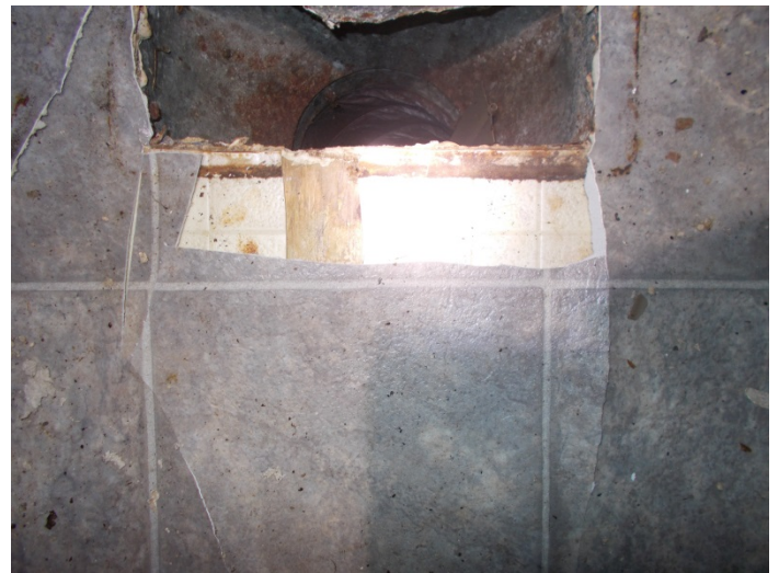
Photo 12 – Stone square pattern vinyl floor with no mastic over cream vinyl floor with mastic.
