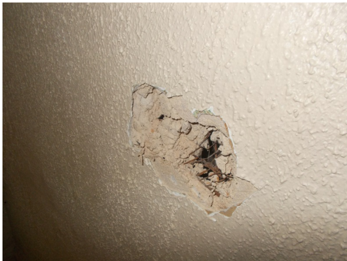
Photo 11 – Texture over plaster with finish throughout the ceilings and walls.
