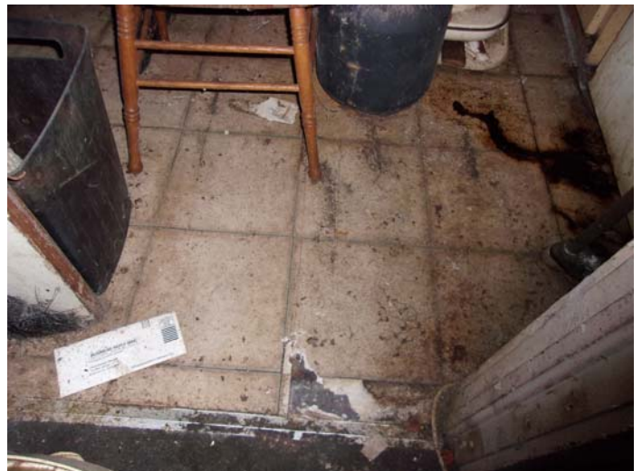
Photo 6 – 12" x 12" beige square pattern self-stick floor tile over light grey vinyl floor & mastic in the kitchen
