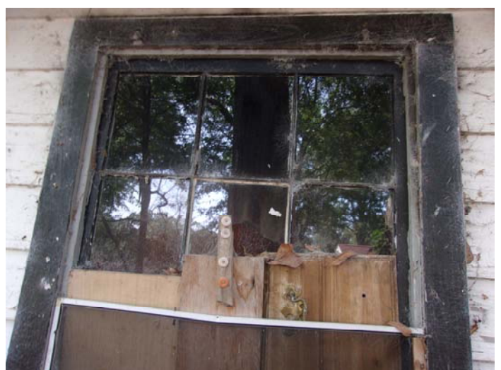
Photo 4 – Wooden windows with glazing
