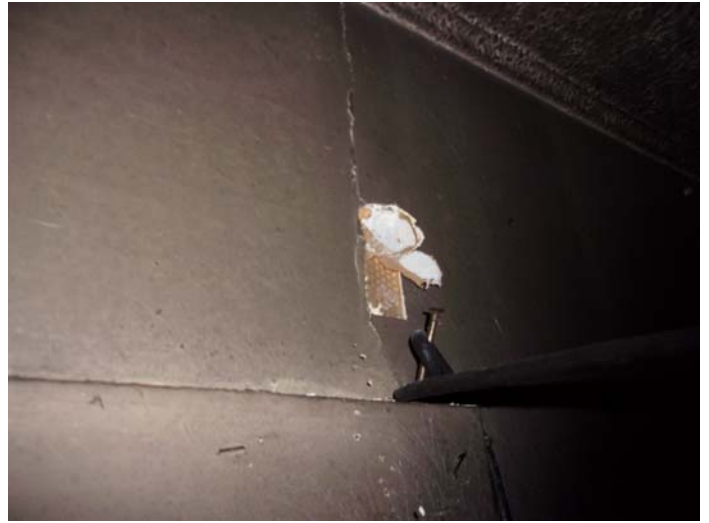
Photo 8 –Drywall with joint compound & tape throughout
