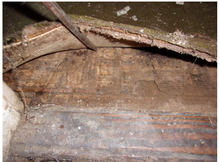
Photo 6 – 2 layers of vinyl floor under carpet in the dining room
