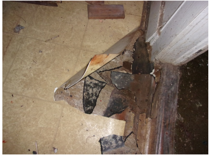
Photo 2 – 5 layers of vinyl flooring in the kitchen
