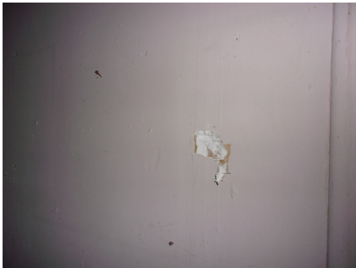
Photo 5 – Drywall with joint compound & tape throughout
