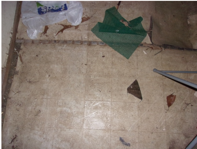
Photo 3 – Tan square pattern vinyl floor with no mastic in the front left room off of the kitchen entry door
