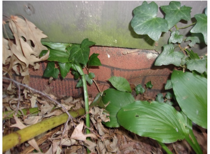
Photo 8 – Red brick pattern roll shingle exterior siding
