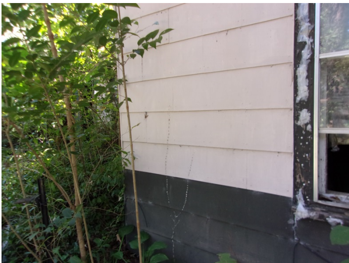
Photo 9 – Cement board exterior siding over felt paper
