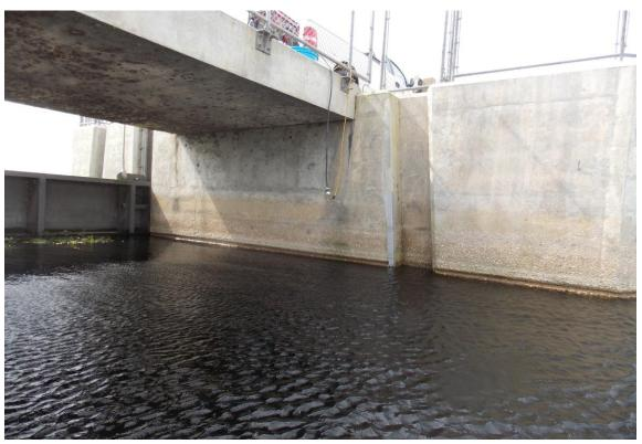
Downstream -South Structure Wall. Note Pitting and "Groove" at Normal Water Level.
