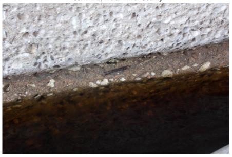
Downstream - South Structure Wall. Note Exposed Steel Reinforcment in "Groove".
