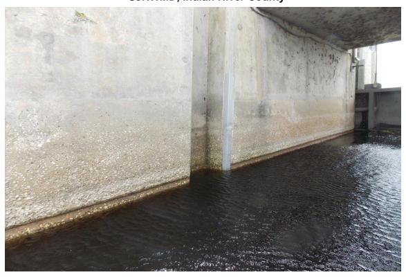
Downstream - North Structure Wall. Note Pitting and "Groove" at Normal Water Level.
