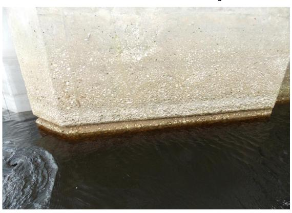
Downstream - North Structure Wall. Note Pitting and "Groove" at Normal Water Level.
