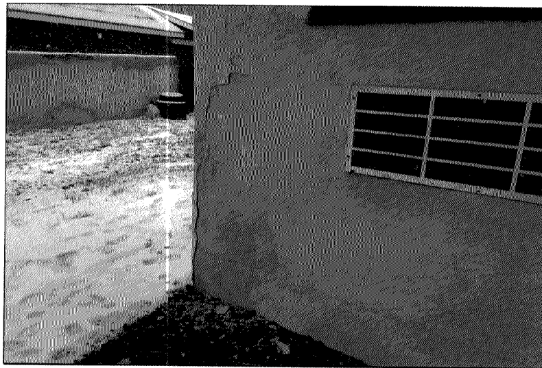
Stucco at Northwest Corner
