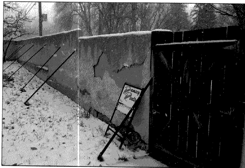
Stucco on Wall
