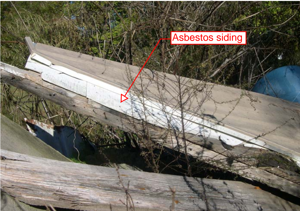
Asbestos contaminated debris pile
