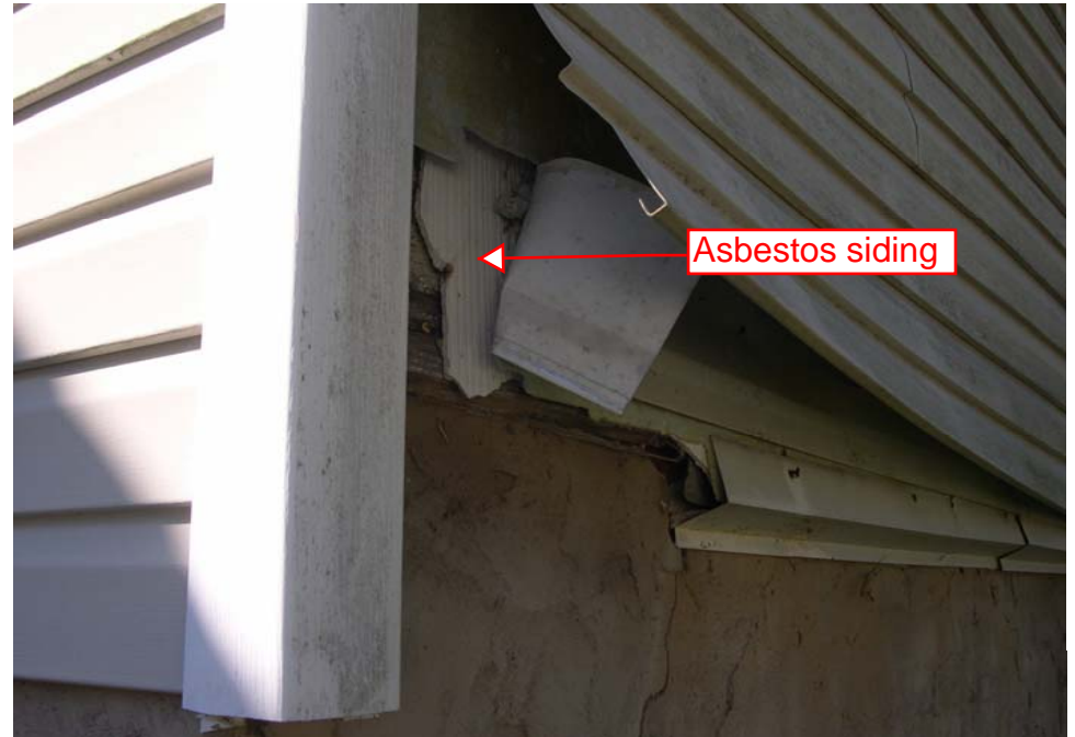
Asbestos exterior siding (transite) under vinyl siding
