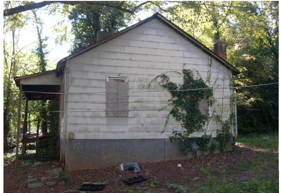
Asbestos exterior siding (transite)
