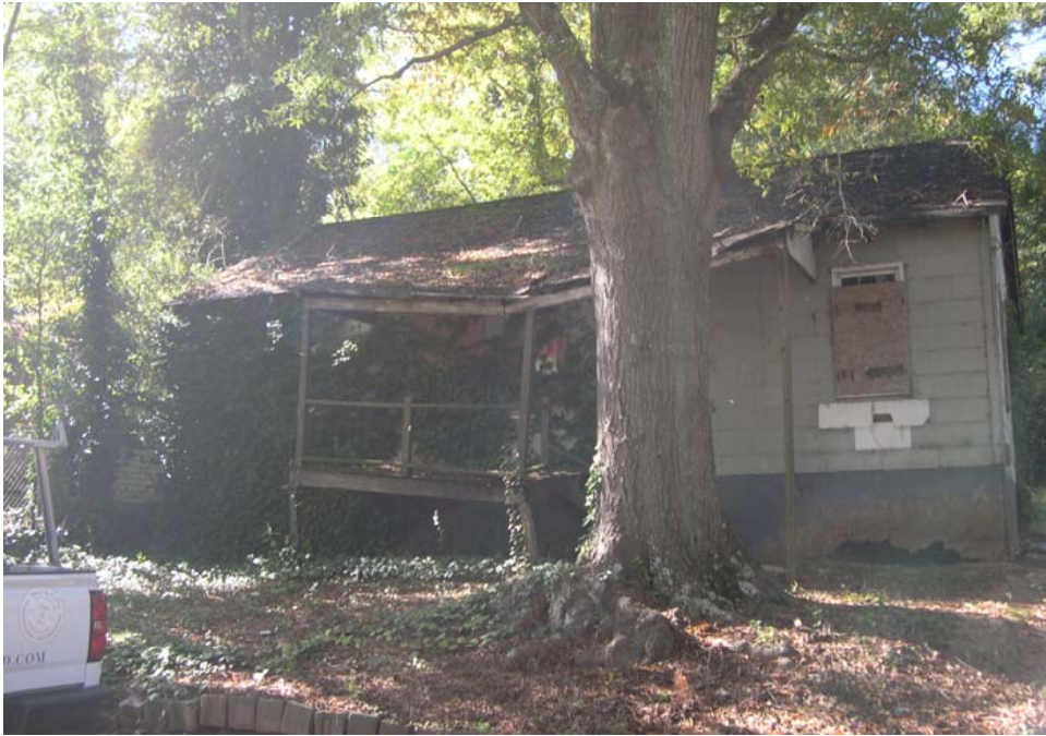
Asbestos exterior siding (transite)
