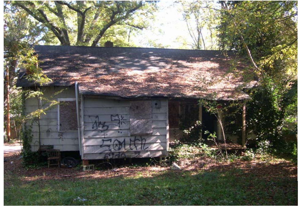
Asbestos exterior siding (transite)
