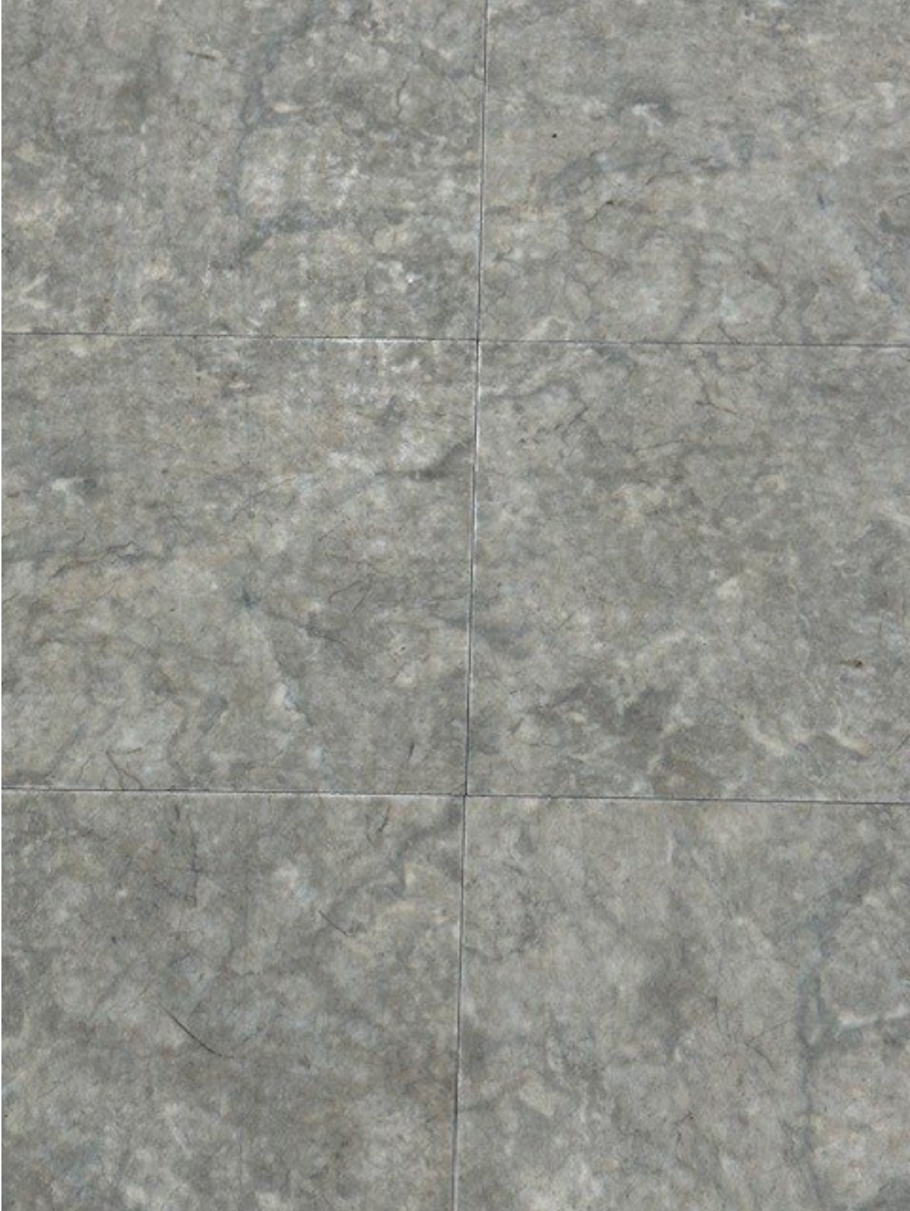
Figure 2: Existing flooring in the Main Hall
