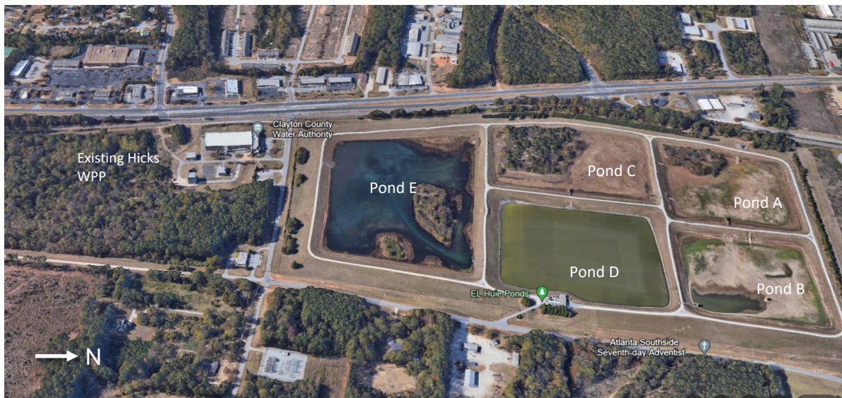
Figure 4-2: Existing Hicks WPP and Huie CTW Ponds
