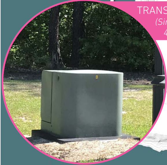
TRANSFORMER (Three-Phase) 110"L x 101"W
