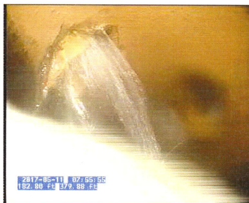
G160 G161_c0caf2a2-9e76-4e62-adbb-02af314ea669.bmp, 00:07:39, 182.84 Infiltration Gusher, at 9 o'clock
