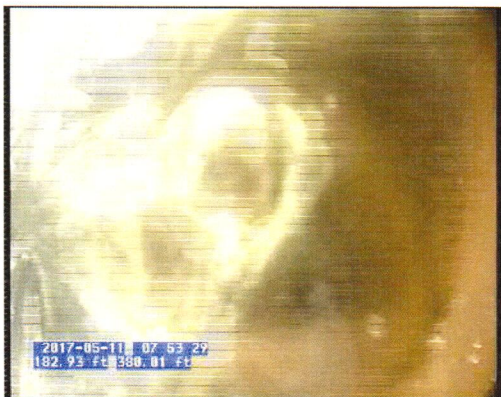
G160 G161_3c4c3644-cfe2-4fd1-ad6b-c565f6a13c6c.bmp, 00:06:31, 182.97 Tap Break-In, at 9 o'clock, 4 inch dim
