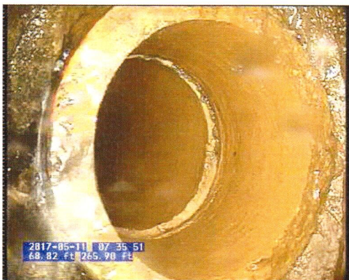
G160 G161_48d84a4b-2377-4ee4-9a3f-ed6f8c312317.bmp, 00:02:08, 68.83 Tap Break-In, at 9 o'clock, 4 inch dim
