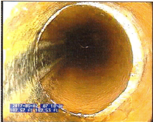
P37 P36_b7094d30-0d4d-454a-88c2-8114f941e086.bmp, 00:05:55, 182.61 Tap Factory Made, at 9 o'clock, 4 inch dim
