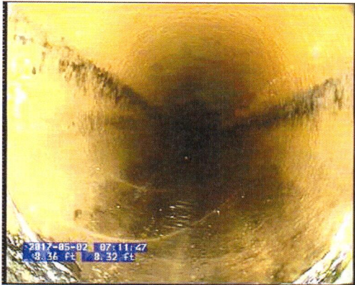
P37P36_2b950ddc-6a67-4b33-93b8-4f85cf56f1a3.bmp, 00:00:17, 8.37 Material Change, Vitrified clay pipe
