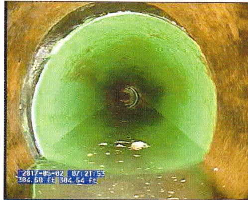
P37 P36_353786e2-1fe4-41bd-b20f-ac543e8f9d10.bmp, 00:08:40, 304.66 Infiltration Runner, at 11 o'clock
