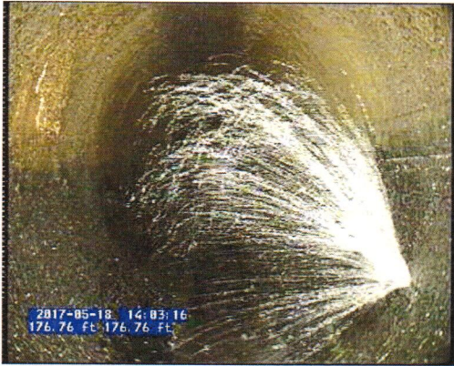
G270 G272_d3e0174d-46f3-4bf9-8d25-161e05baba4b.bmp, 00:03:55, 176.80 Infiltration Gusher, at 4 o'clock
