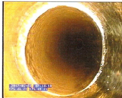
P37P36_7e6232c3-7cf3-427c-9535-e85cba75259d.bmp, 00:05:36, 175.49 Tap Factory Made, at 3 o'clock, 4 inch dim
