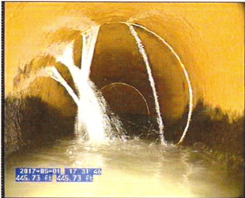
P36 P74 (2)_1d7db7c9-9892-4522-b16b-7c32cfc485b6.bmp, 00:09:07, 445.83 Infiltration Gusher, at 12 o'clock
