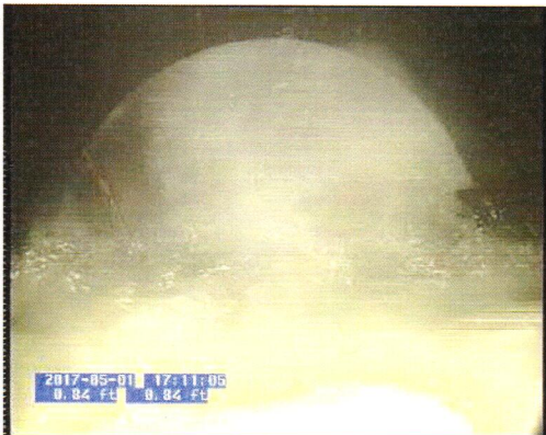
P36 P74_db4e454f-3ba2-473e-9445-4154ee93850e.bmp, NaN:NaN, 1.02 Survey Abandoned, offset joint
