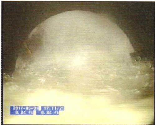
P36 P74_fdd61753-f9be-410f-844d-23e9d200c77e.bmp, NaN:NaN, 1.02 Survey Abandoned, offset joint
