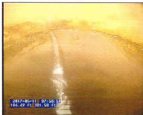
G160 G161_01c89cc4-169b-4891-8b8c-66de64491820.bmp, 00:08:17, 184.55 Infiltration Runner, at 12 o'clock
