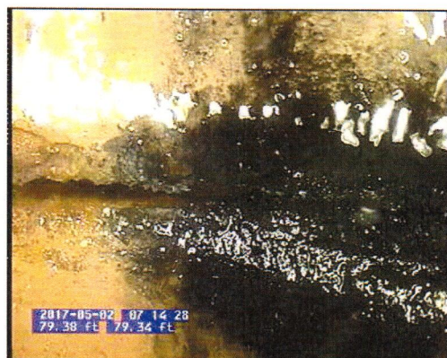
P37P36_6e7177d3-16e3-4271-b7c2-5739d3d25ec2.bmp, 00:02:43, 79.40 Infiltration Weeper, at 4 o'clock
