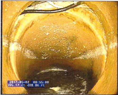
P86 P36_6c59f69c-2e0f-43af-9dd0-b94bcb7fe39a.bmp, 00:05:23, 285.24 Joint Offset Large, 0 ° displacement
