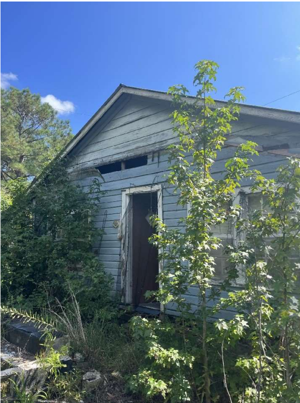
Exterior Front Door
