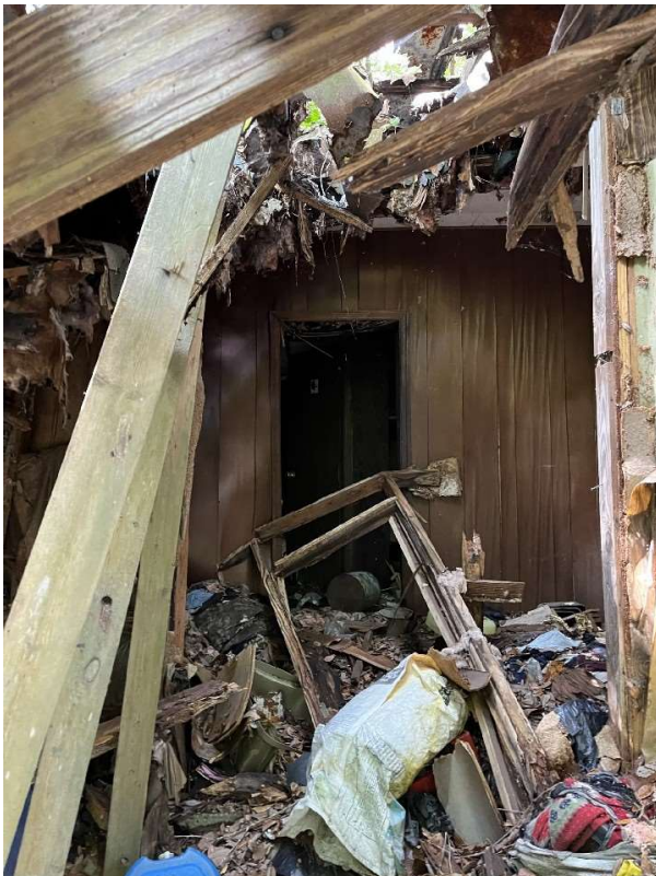
Interior Rear Addition
