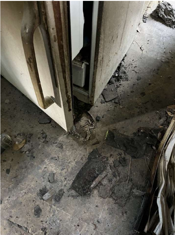
Interior Kitchen Floor
