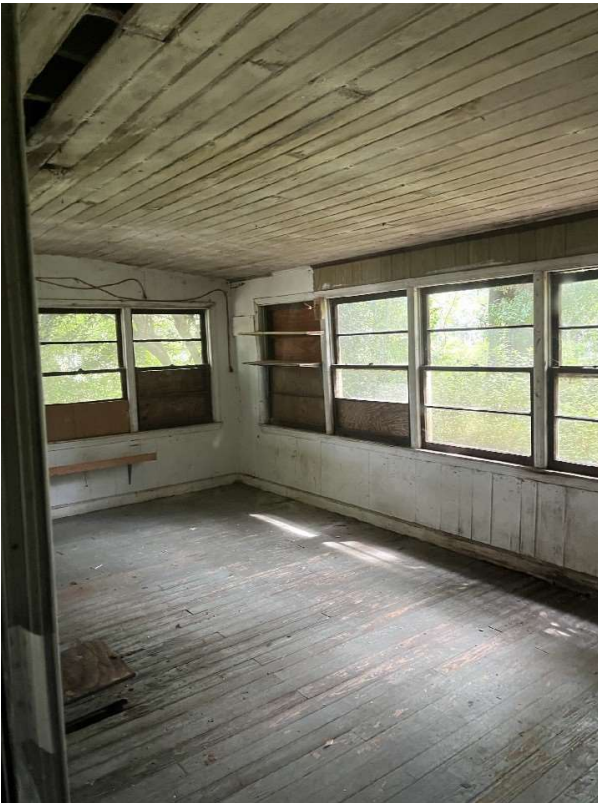
Interior Front Porch
