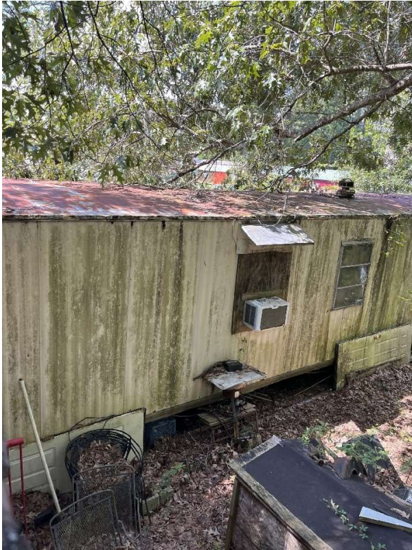
Exterior Roof of Mobile Home
