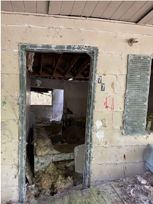
Exterior Front Door
