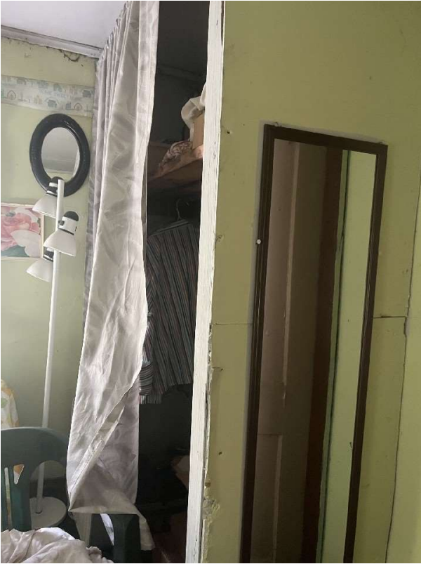
Interior Left Rear Bedroom Closet
