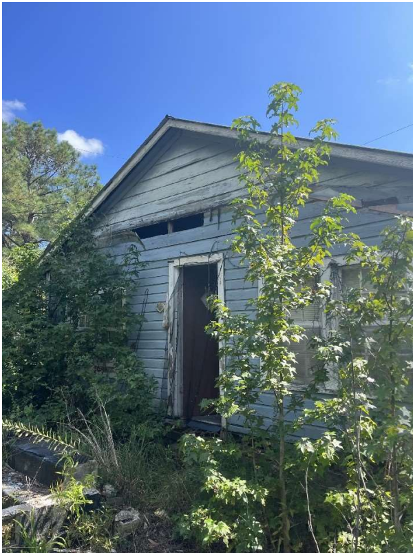
Exterior Front Door Area
