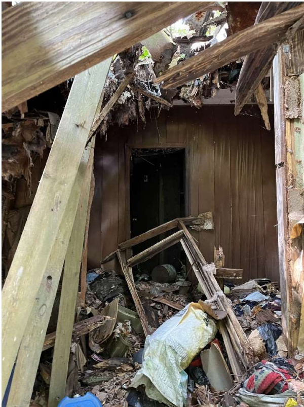
Interior Rear Addition
