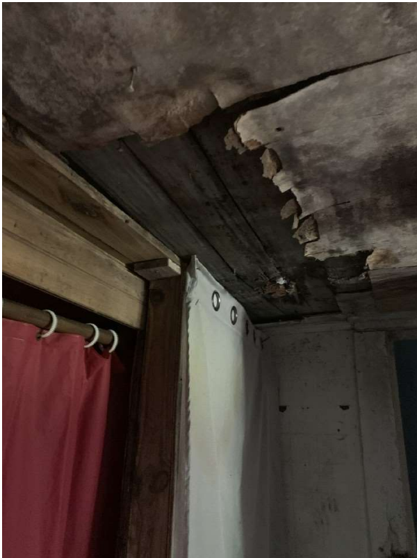
Interior Bathroom Ceiling
