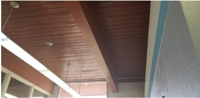
Figure 23: INTERIOR WOOD AND GLULAM BEAM FRAMING – PASSENGER WAITING AREA
