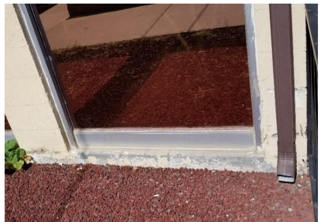
Figure 25: EXTERIOR NW STEM WALL AT VESTIBULE
