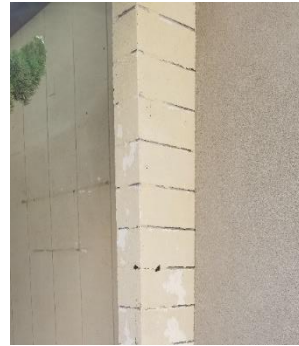
Figure 22: EXTERIOR CMU COLUMN
