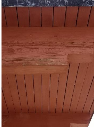
Figure 21: EXTERIOR GLULAM BEAM – WEATHERED DETAIL
