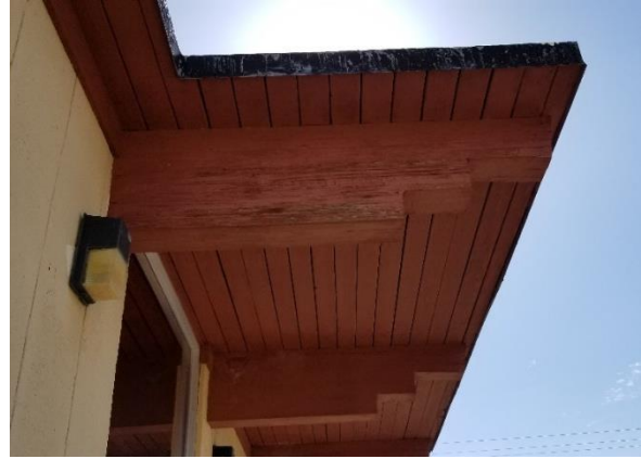
Figure 20: EXTERIOR GLULAM BEAM
