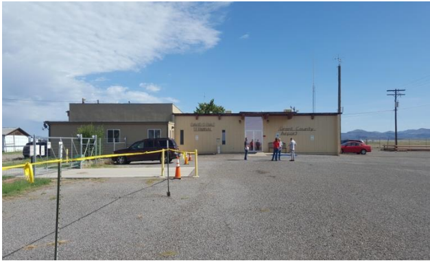
Figure 12: P1 SOUTH VIEW
