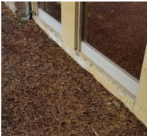
Figure 24: EXTERIOR NW STEM WALL AT VESTIBULE
