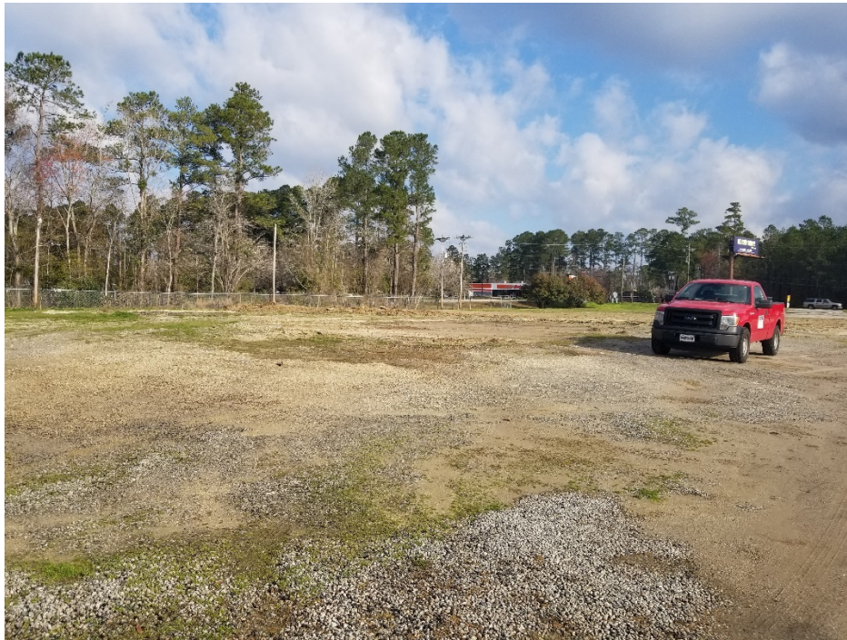
Figure 4: Looking Northwest from Southeast Corner
