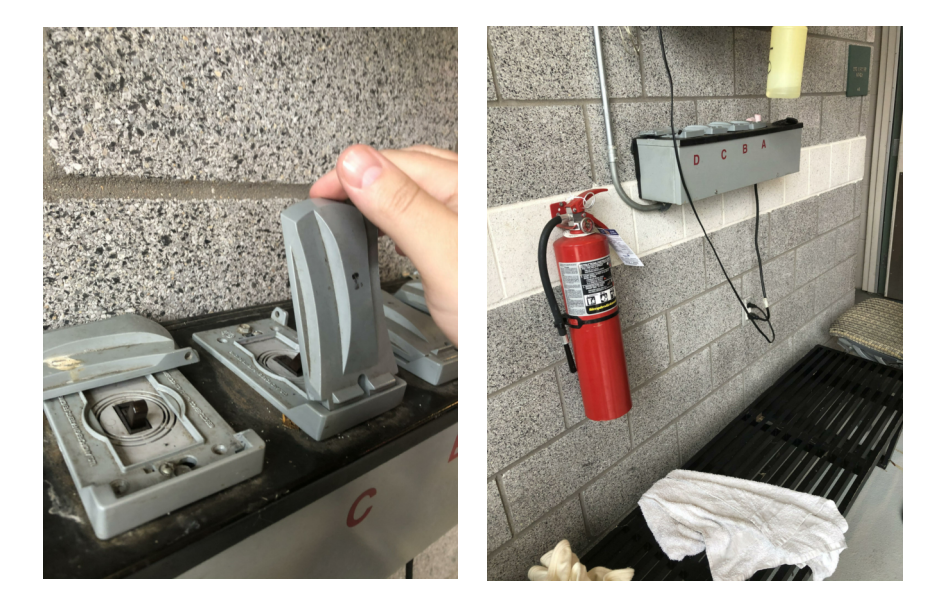
RELOCATE HOSE REEL SOLENOID SWITCH ASSEMBLY
