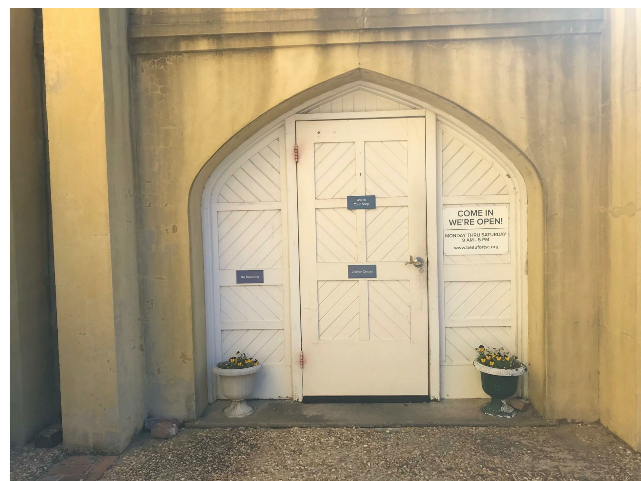
EXISTING CONDITIONS- ACCESS DOOR 1 EXTERIOR NOT TO SCALE
