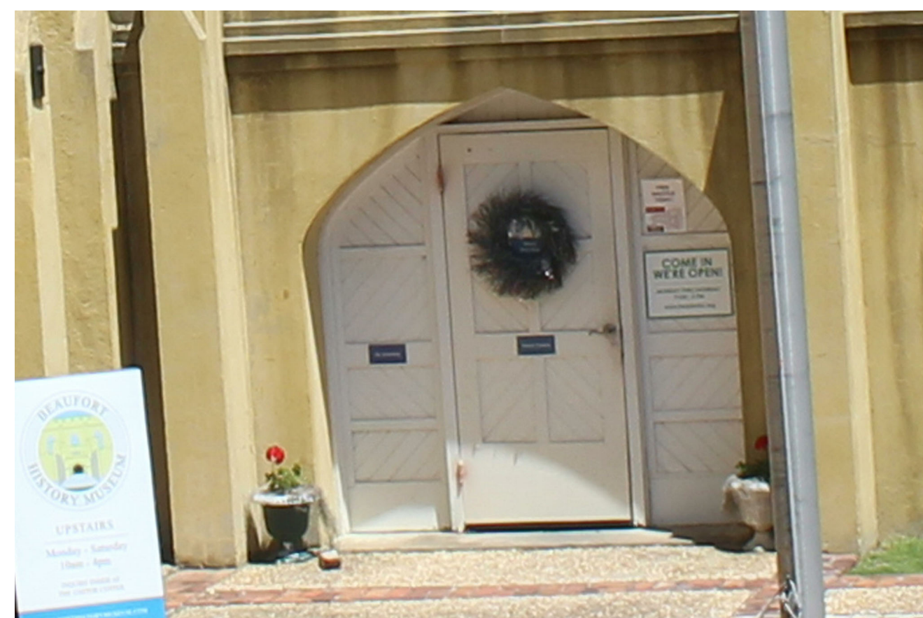
EXISTING CONDITIONS- ACCESS DOOR 2 EXTERIOR NOT TO SCALE
