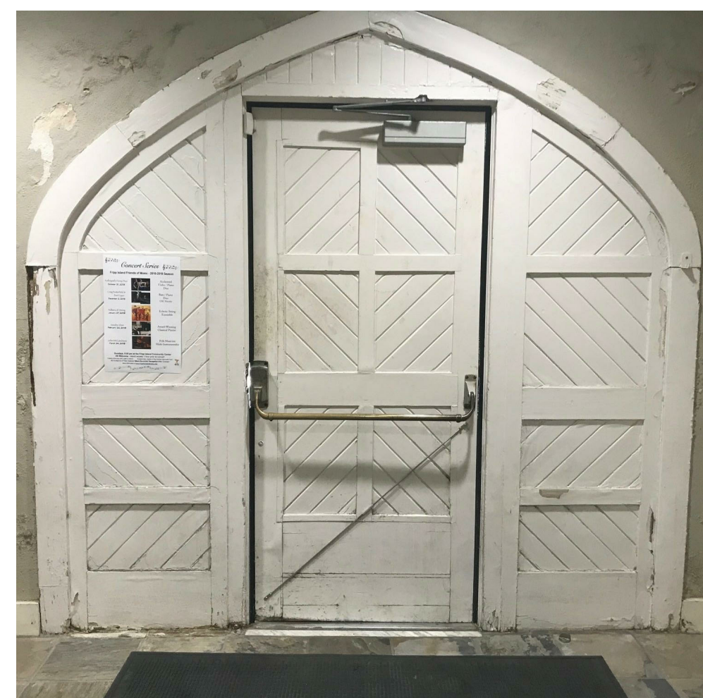
EXISTING CONDITIONS- ACCESS DOOR 1 INTERIOR NOT TO SCALE
