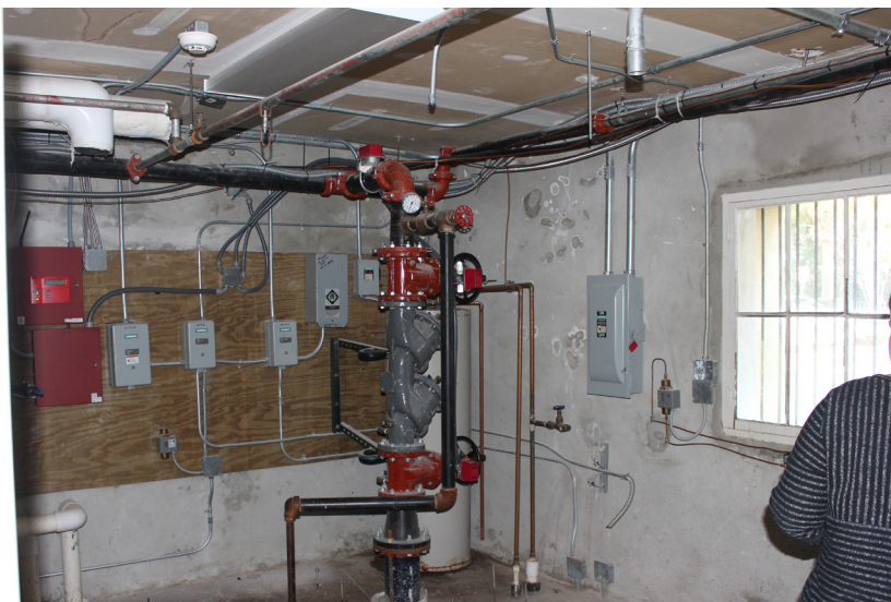
Figure 85: Detail of interior conditions.
