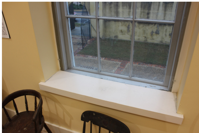
Figure 25: Detail of interior conditions.
