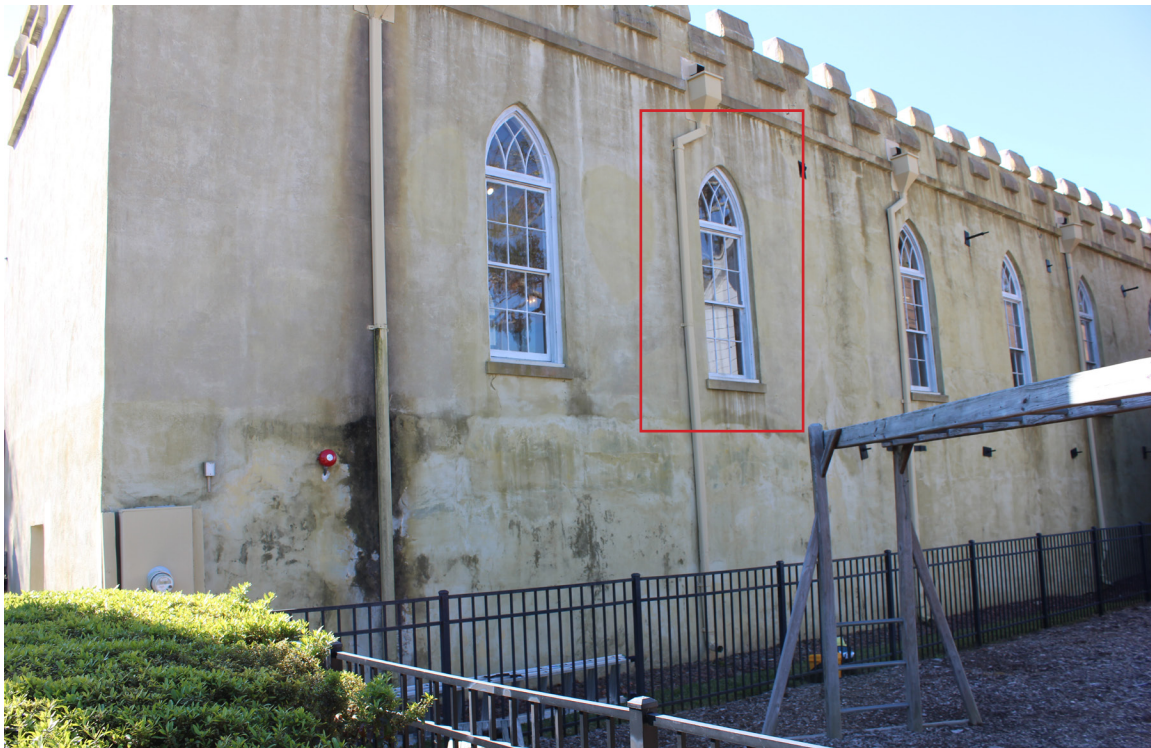
Figure 90: Overview of window #W-21. This is an historic double-hung sash window.
