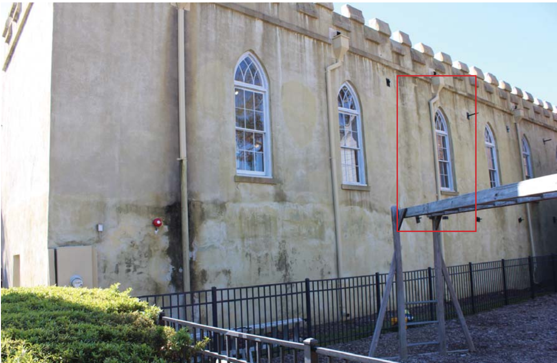
Figure 94: Overview of window #W-22. This is an historic double-hung sash window.
