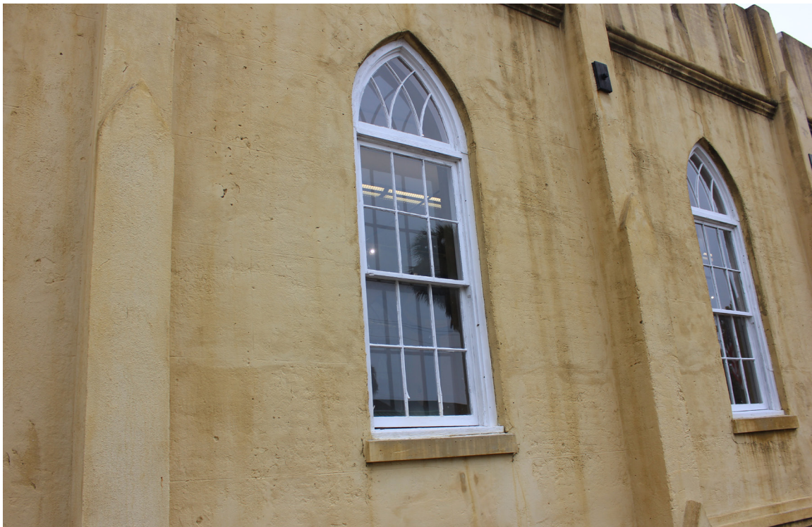
Figure 18: Overview of window #W-03. This is an historic double-hung sash window.
