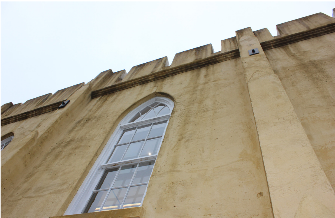
Figure 26: Overview of window #W-05. This is an historic double-hung sash window.
