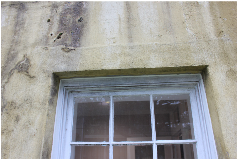
Figure 159: The wooden elements are in good condition.
