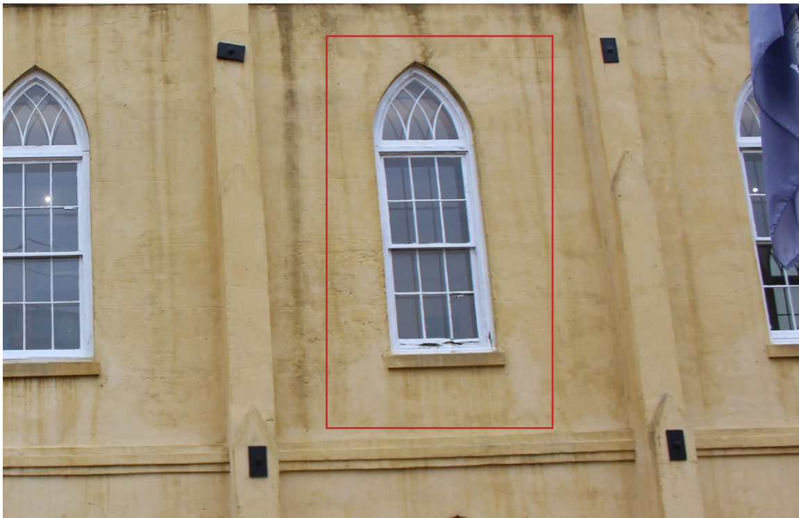
Figure 34: Overview of window #W-07. This is an historic double-hung sash window.
