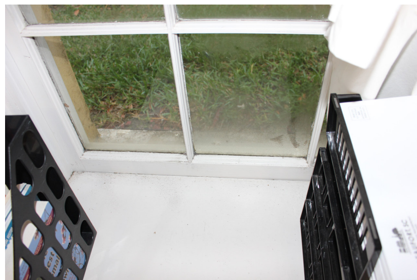
Figure 73: Detail of interior conditions.
