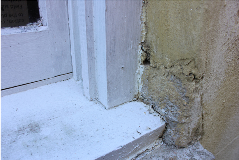
Figure 116: Detail of stucco repair.
