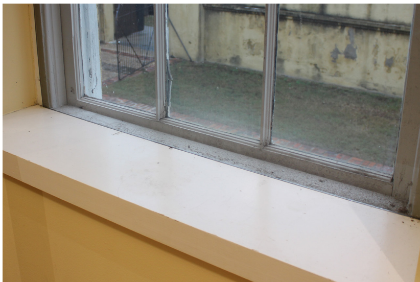
Figure 21: Detail of interior conditions.
