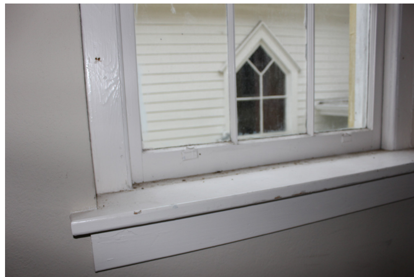
Figure 125: Detail of interior conditions.
