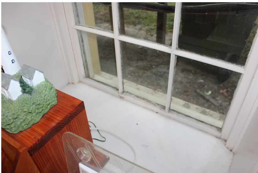
Figure 81: Detail of interior conditions.
