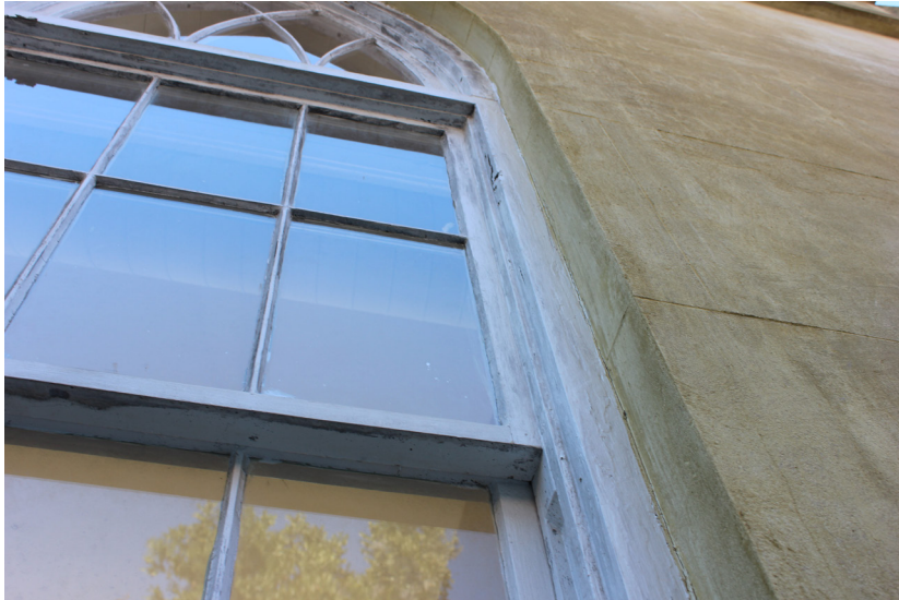
Figure 124: The casing and frame are in good condition.
