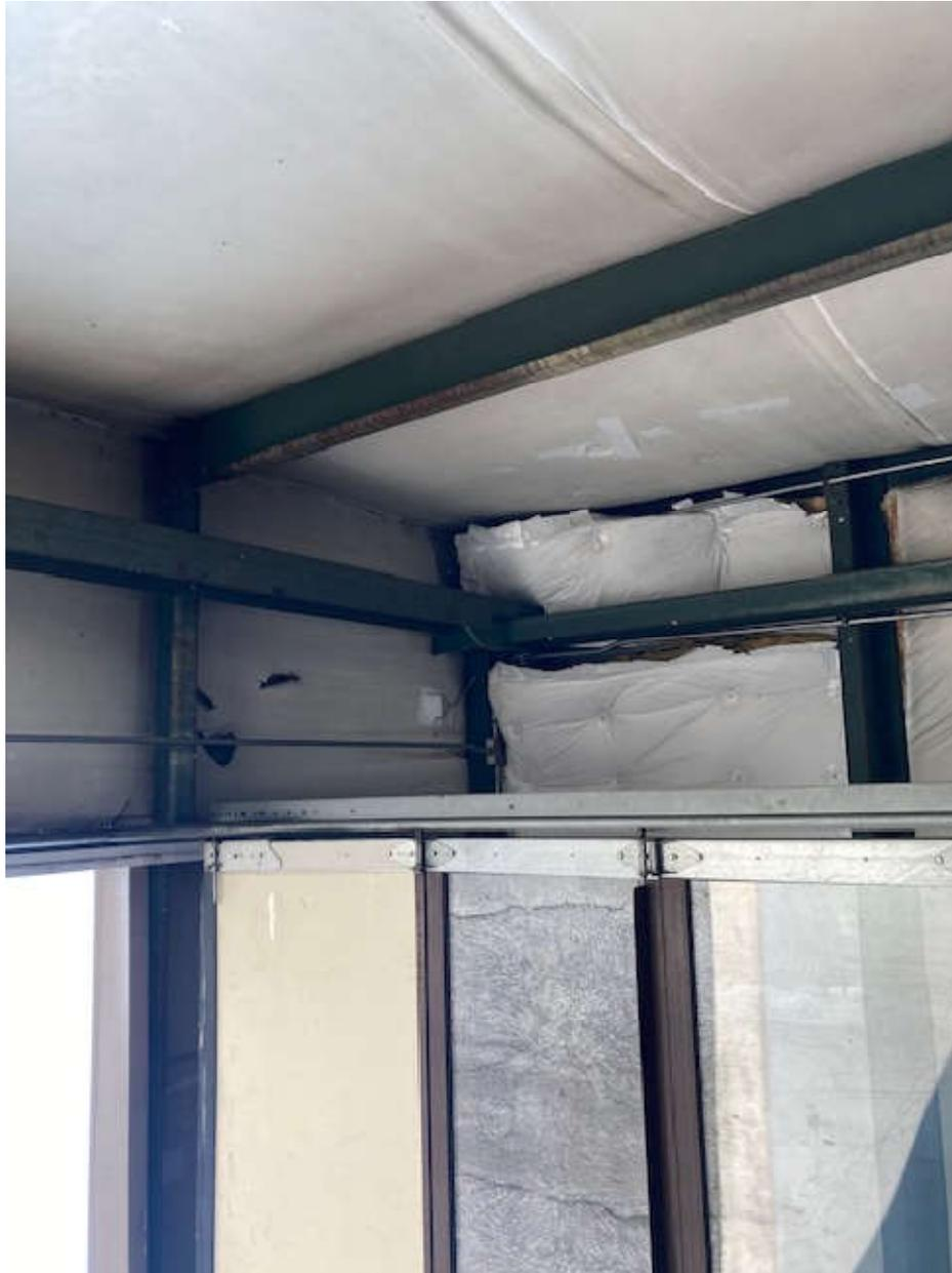
Deteriorated Insulation at Previous Roof Leak Point
