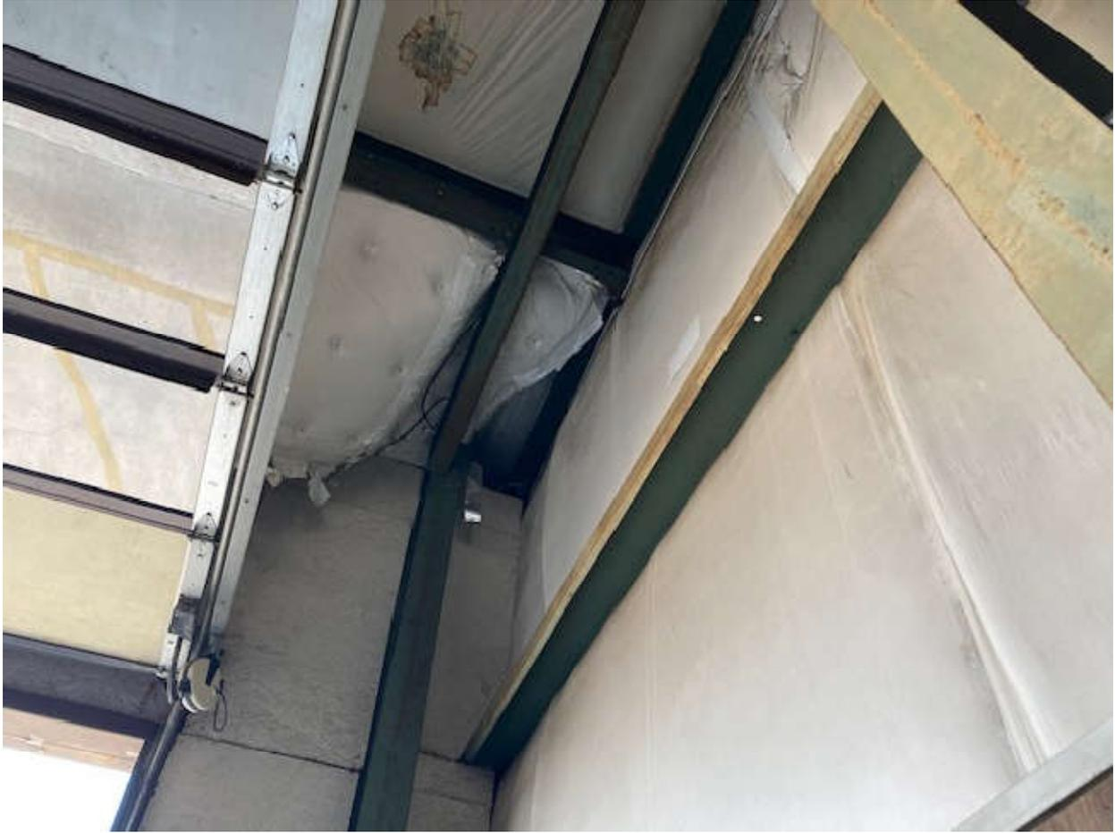
Deteriorated Insulation at Previous Roof Leak Point
