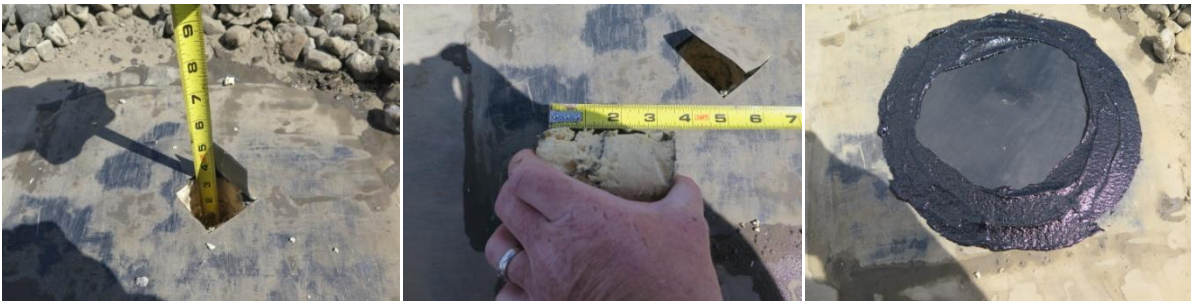
Core #2 – Metal Deck, 3" ISO, Ballasted EPDM - Dry
