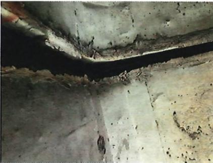
Figure 4: Separated joint
