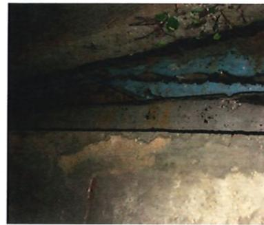
Figure 2: Soil infiltration due to leaked joint 2
