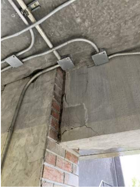
PHOTO 49: CRACKING AT SOUTH END OF BEAM ADJACENT TO STAIRS
