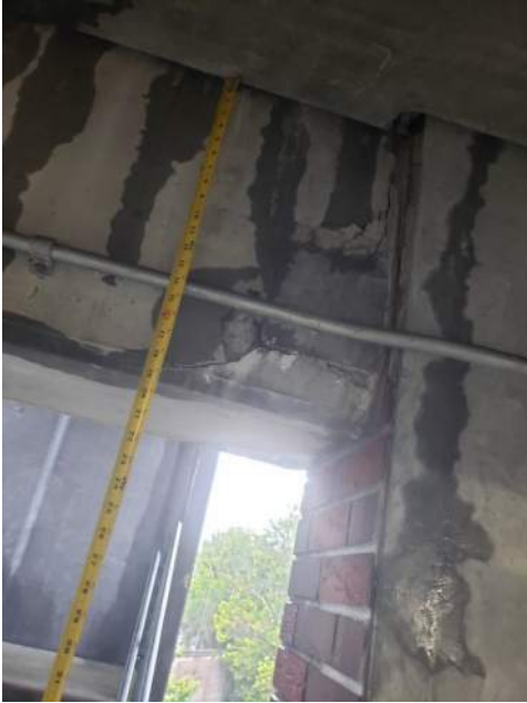
PHOTO 46: CRACKED AND SPALLED CONNECTION AT NORTH END OF LANDING BEAM
