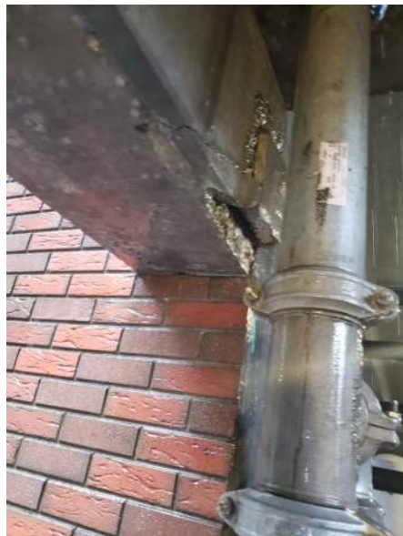
PHOTO 36: CRACKING AND SPALLING AT SOUTH END OF LANDING BEAM
