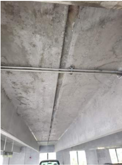
PHOTO 17: TAPERED JOINT BETWEEN PRECAST DOUBLE-TEE MEMBERS
