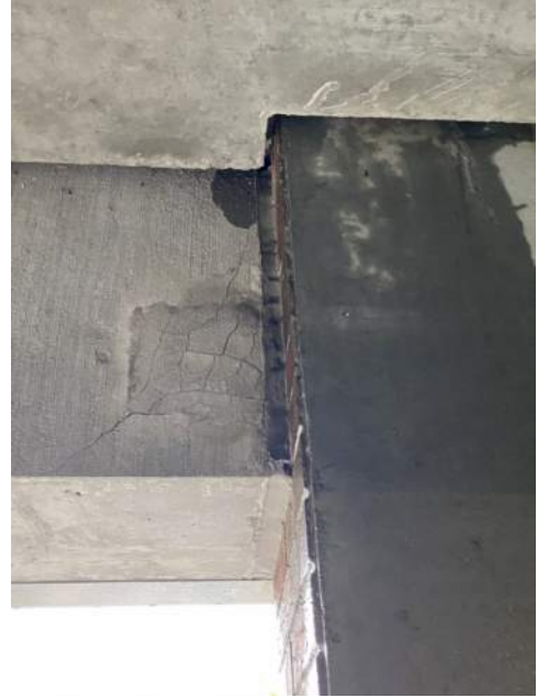
PHOTO 49: CRACKING AT SOUTH END OF BEAM ADJACENT TO STAIRS
