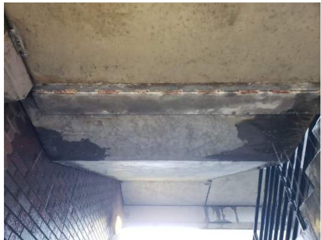
PHOTO 30: CORROSION AT STAIR FLIGHT CONNECTIONS TO LANDING BEAM
