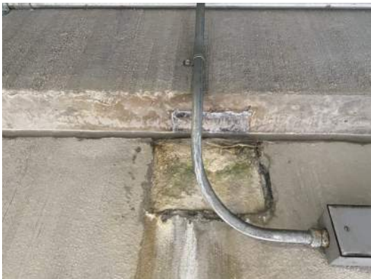
PHOTO 51: SPALLED CONNECTION AT INT. SUPPORT OF BEAM ADJACENT TO STAIRS
