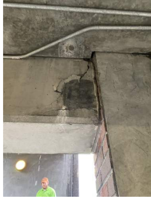
PHOTO 46: CRACKED AND SPALLED CONNECTION AT NORTH END OF LANDING BEAM
