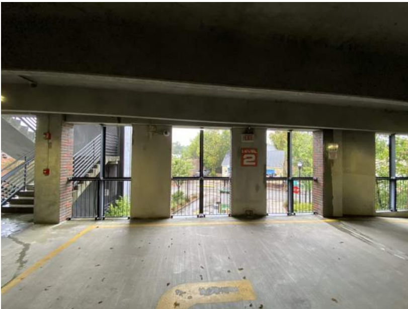
PHOTO 48: BEAM LINE ADJACENT TO STAIRS
