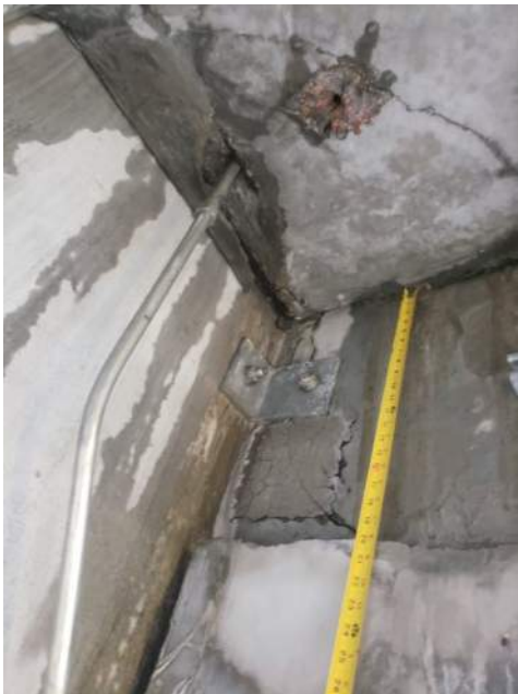
PHOTO 44: CRACKED AND SPALLED CONNECTION AT SOUTH END OF LANDING BEAM
