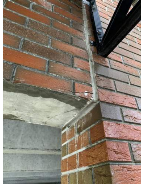
PHOTO 53: CRACKING AT SOUTH END OF BEAM OVER MAIN GARAGE ENTRANCE
