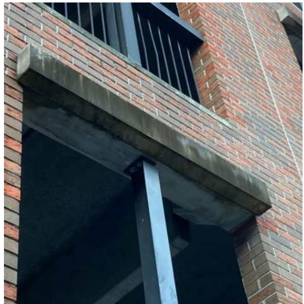
PHOTO 3: MOISTURE AND ORGANIC GROWTH ON CAST STONE PIECES
