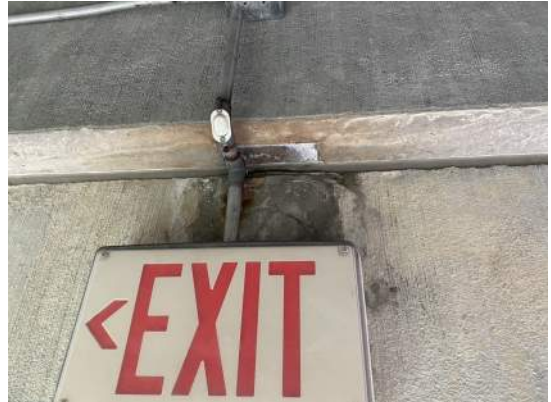
PHOTO 51: SPALLED CONNECTION AT INT. SUPPORT OF BEAM ADJACENT TO STAIRS
