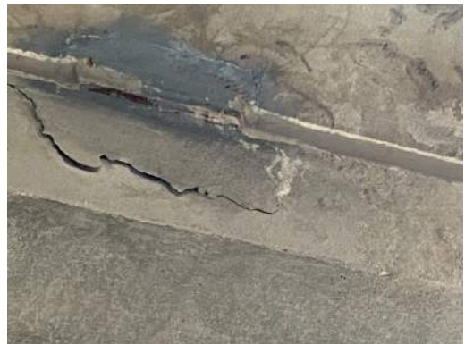
PHOTO 42: SPALLED AND CORRODED LANDING SLAB CONNECTION TO CORBEL
