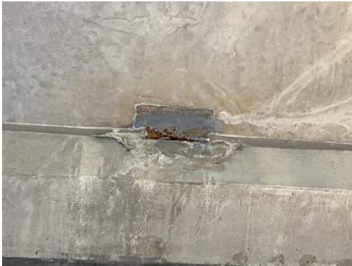
PHOTO 42: SPALLED AND CORRODED LANDING SLAB CONNECTION TO CORBEL
