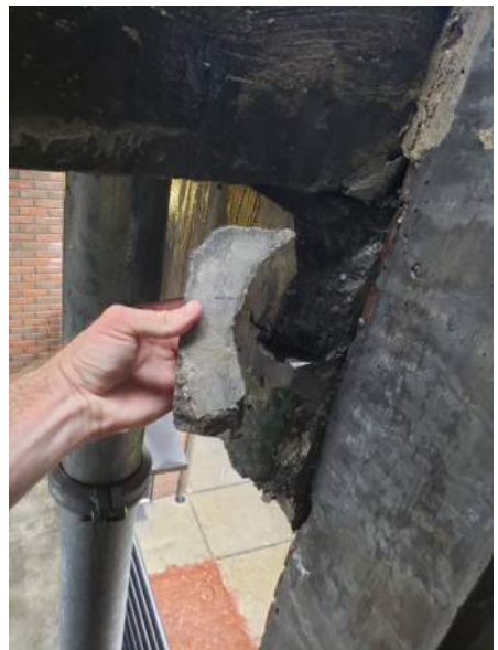
PHOTO 36: CRACKING AND SPALLING AT SOUTH END OF LANDING BEAM
