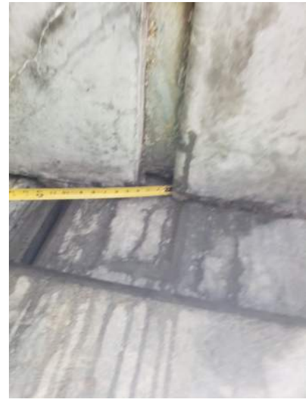
PHOTO 17: TAPERED JOINT BETWEEN PRECAST DOUBLE-TEE MEMBERS
