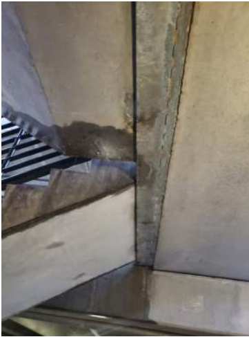
PHOTO 30: CORROSION AT STAIR FLIGHT CONNECTIONS TO LANDING BEAM
