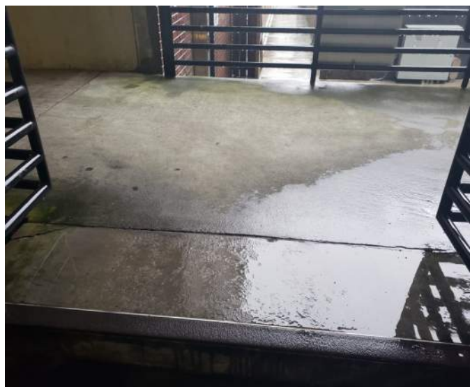
PHOTO 24: RAINWATER RUNOFF THROUGH STANDPIPE OPENING
