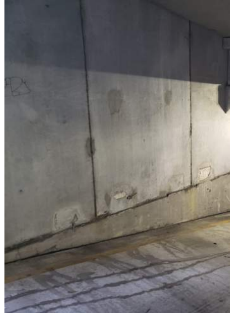
PHOTO 13: SPALLED INTERMEDIATE LEVEL PANEL CONNECTION
