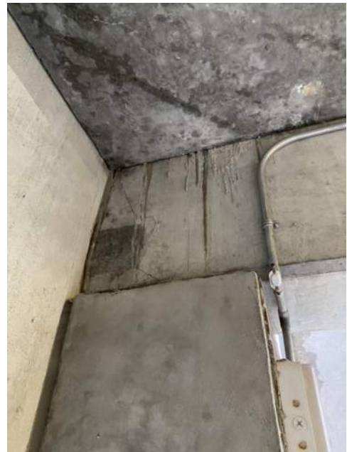
PHOTO 44: CRACKED AND SPALLED CONNECTION AT SOUTH END OF LANDING BEAM
