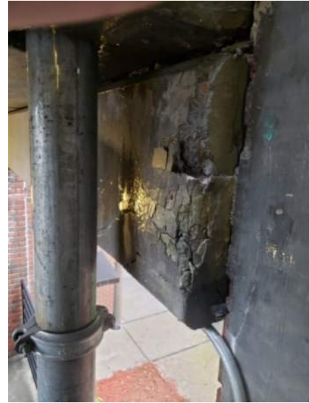
PHOTO 34: CRACKING AND SPALLING AT SOUTH END OF LANDING BEAM
