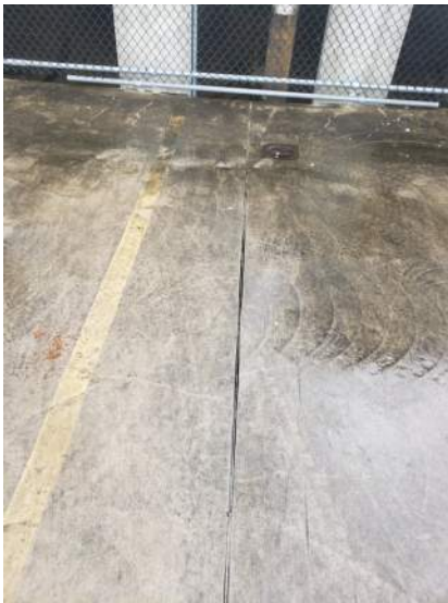
PHOTO 7: TOPPING SLAB JOINT AT UPPER LEVEL DECK
