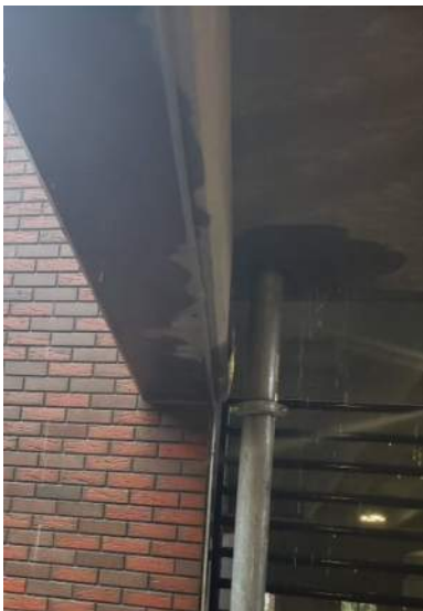
PHOTO 24: RAINWATER RUNOFF THROUGH STANDPIPE OPENING
