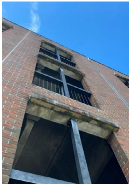
PHOTO 3: MOISTURE AND ORGANIC GROWTH ON CAST STONE PIECES
