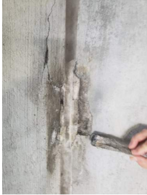
PHOTO 13: SPALLED INTERMEDIATE LEVEL PANEL CONNECTION
