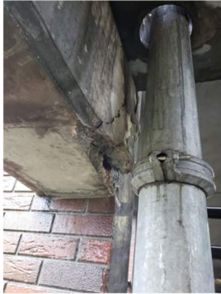
PHOTO 34: CRACKING AND SPALLING AT SOUTH END OF LANDING BEAM
