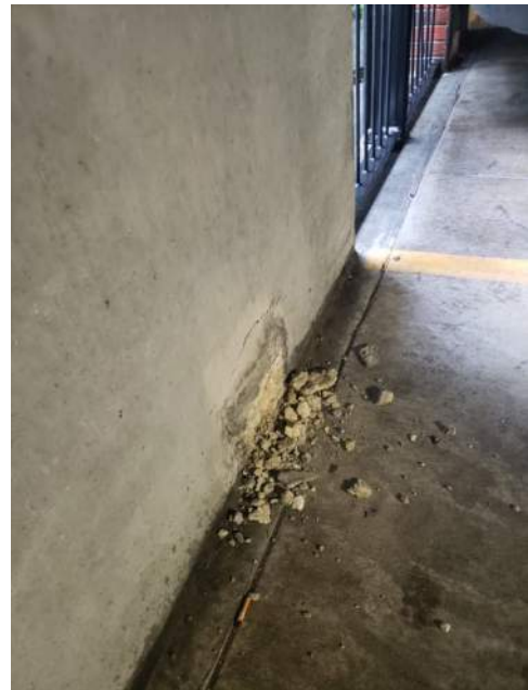
PHOTO 15: EXPANSIVE SPALLING GROUT AT WALL PANEL BASE CONNECTION
