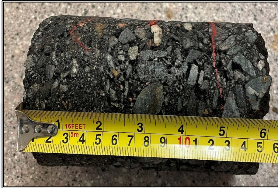
Sample #BH30 (Riverside Drive)
